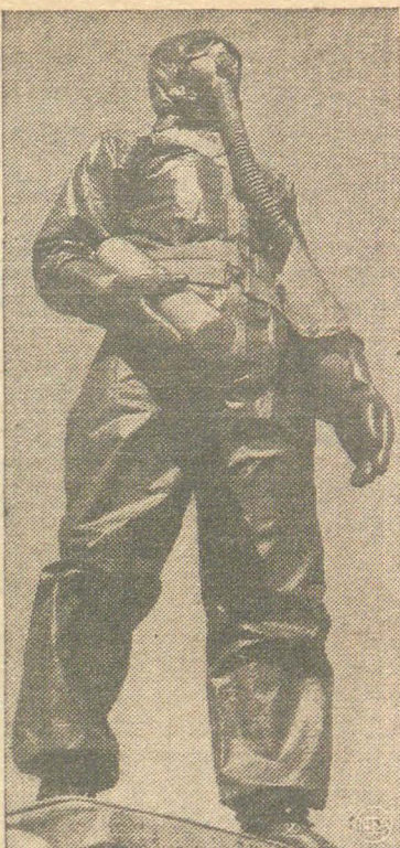
Suit worn by Warren Gromberg, Tarrant Field, Tex., isn't a Thing to Come; it's really here. The rubberized gear is used for decontaminating gassed areas and equipment.
