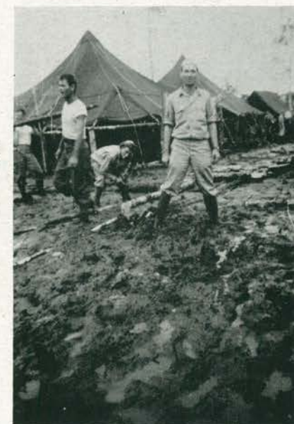
Probably the messiest job we had was to remove tree roots and rotten logs from this ooze, so that the tent areas could be drained and walks built.
