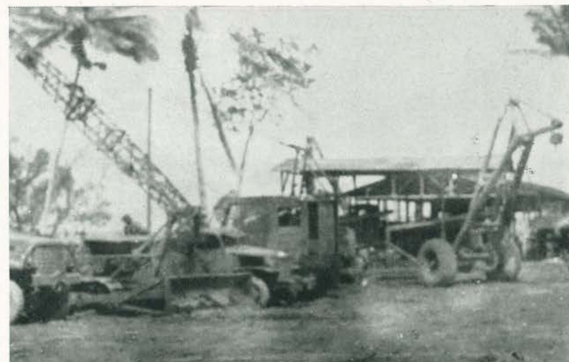
The A-frame at right was used to transfer barge sections around the area.
