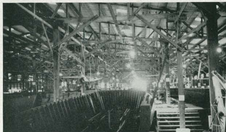
After the external hull is complete, the boat is rotated, and work starts on the interior. Above, the flooring is being laid
