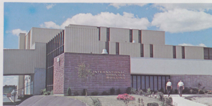
New international arrivals building in Bangor
