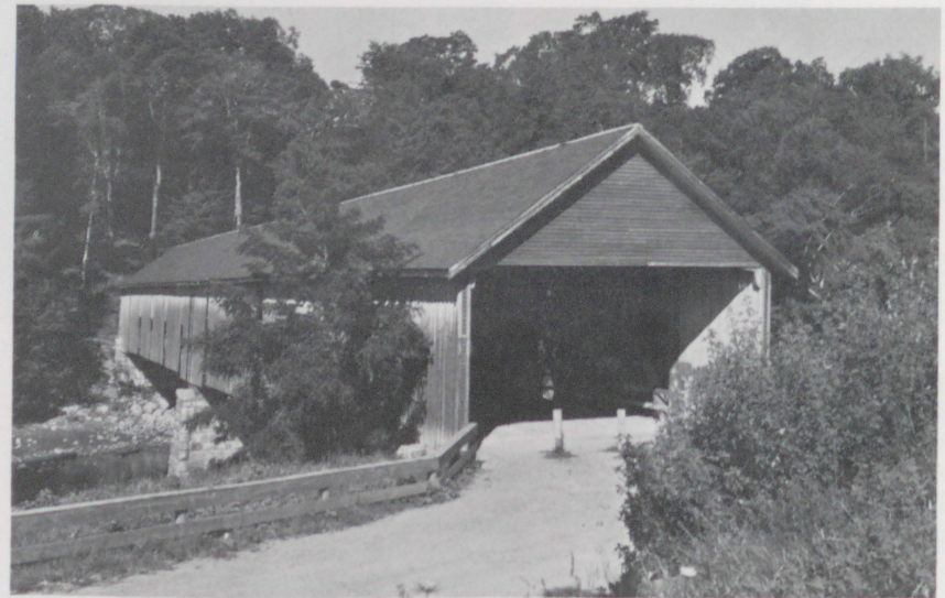
Morse Covered Bridge spans the Kenduskeag Stream.
