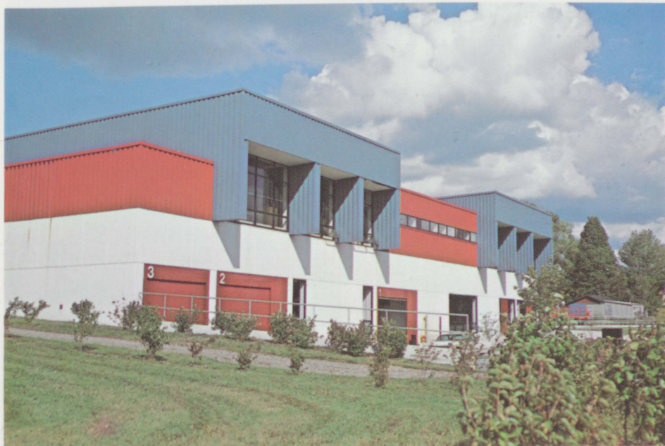
Brewer's modern waste water treatment plant
