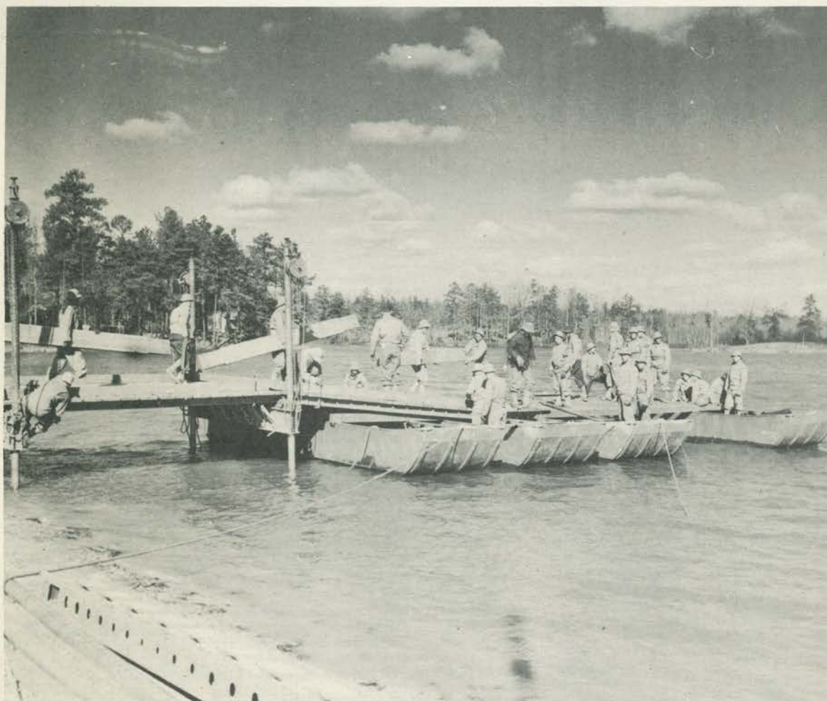
Ponton bridge construction at Birchen Lake
