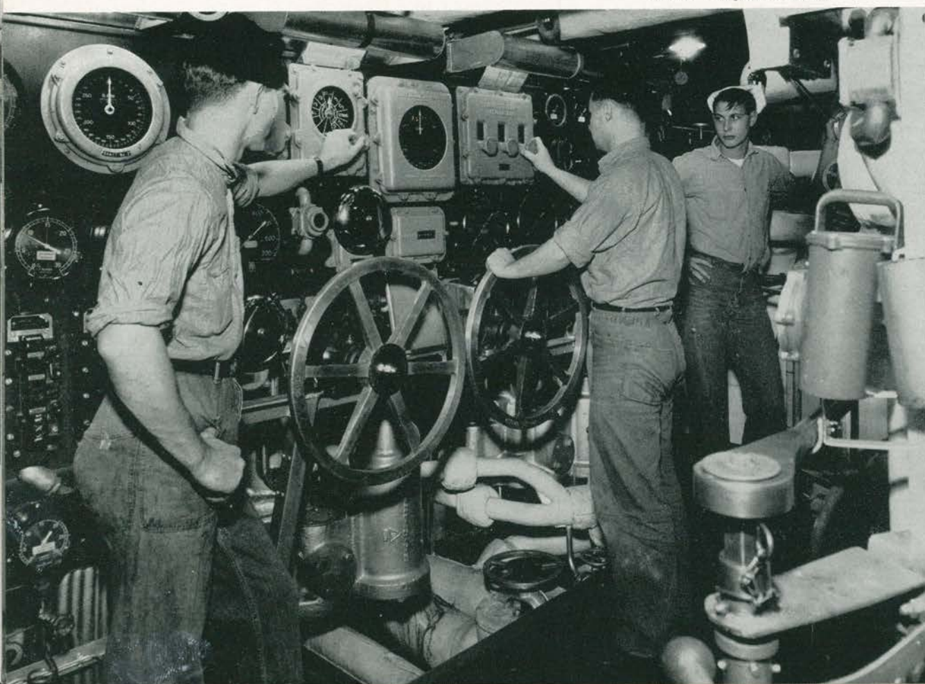
Main Engine Room
