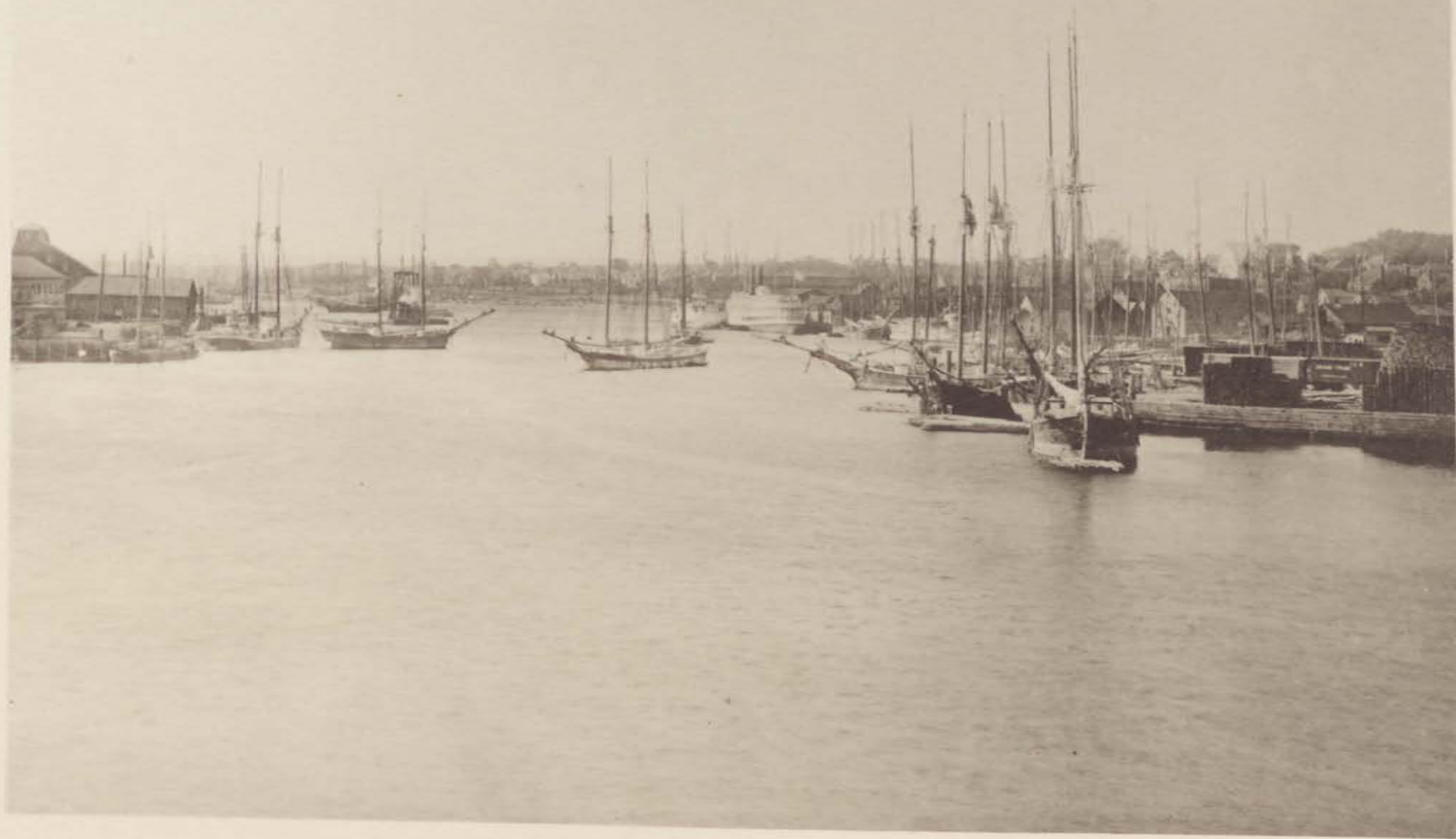
VIEW OF PENOBSCOT RIVER FROM THE BRIDGE.
