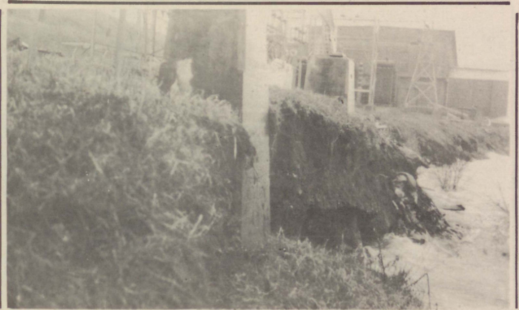
High water in Forebay at Veazie Station, showing outside wall of Generator Room. Platform which runs entire length of station used for track for rack rake under water.
