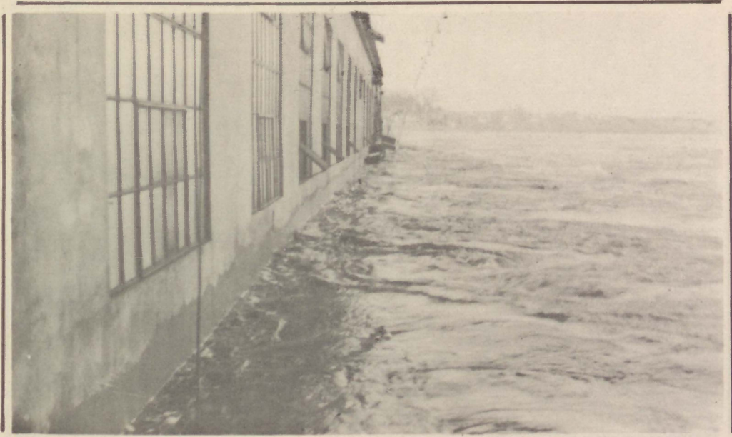
High water in Forebay at Veazie Station, showing outside wall of Generator Room. Platform which runs entire length of station used for track for rack rake under water.
