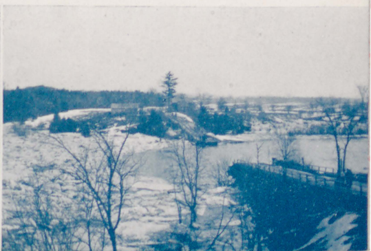
Dudley Bridge Site—Afterwards
