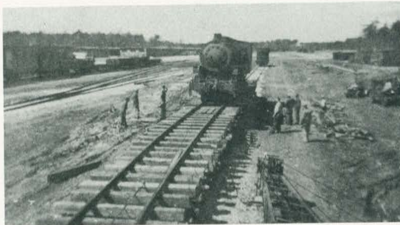
We build a ramp
