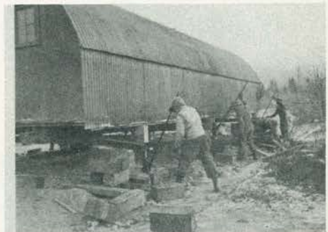
Raising Quonset for the trailer
