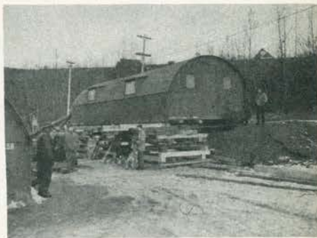
Going in place
