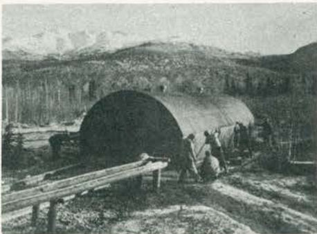
Digging a Quonset out of the frozen ground
