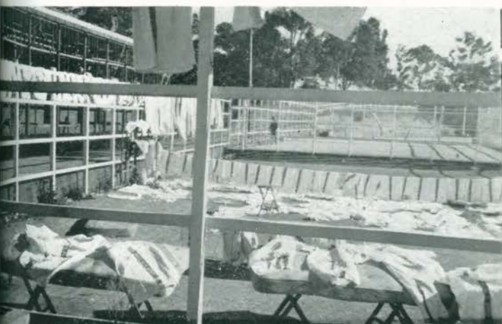
Drying salvaged goods from the "Rufus King."
