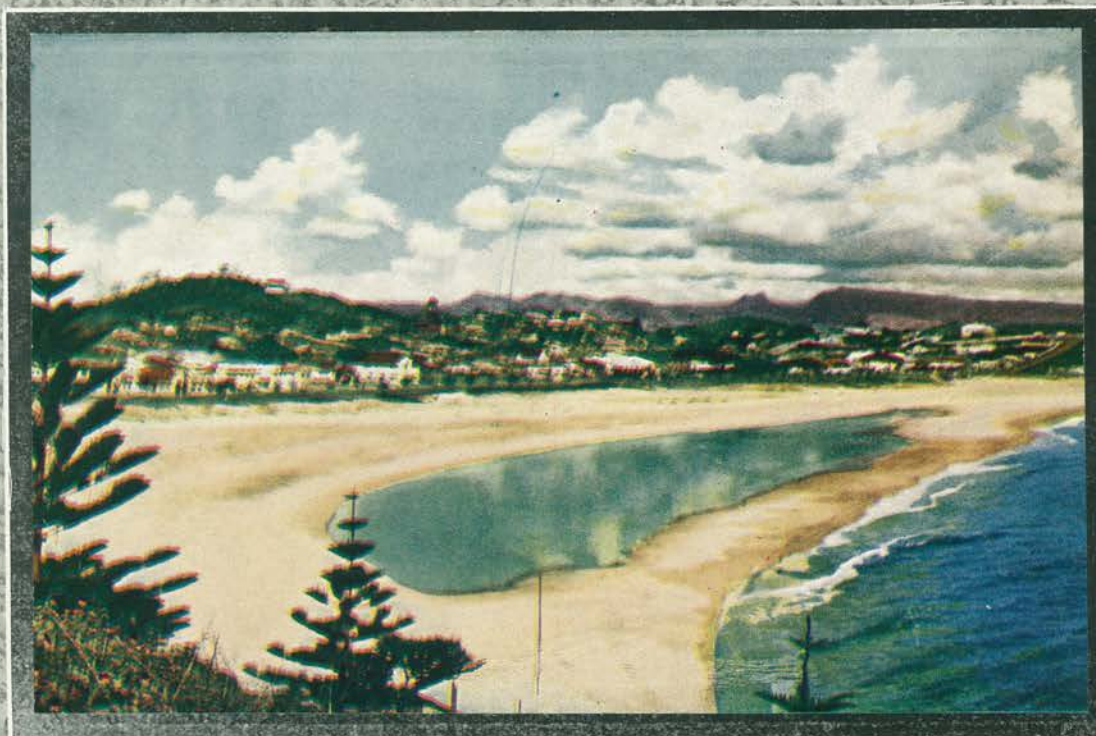
Coolangatta looking from Greenmount
