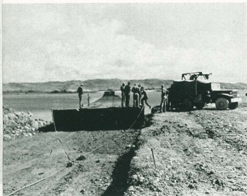
One end of the pontoon assembly was pulled ashore by a "cat"
