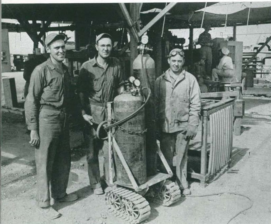
★ Seidenberg, Wyatt and Garrison put junkyard caterpillar rollers from an old bomb carrier on to a field welding tank so that it could be pushed easily over the roughest terrain.
