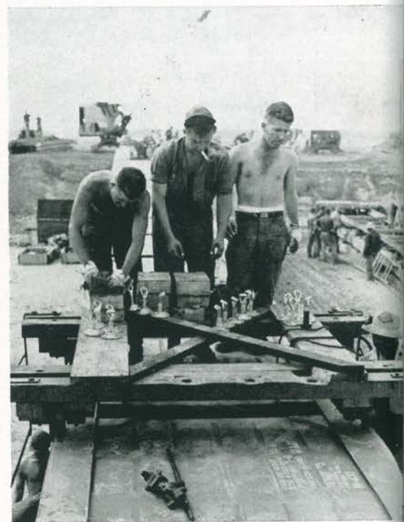
Stokey, Stackhouse and Sharp set up the "Toonerville Trolley" which Sharpe had designed to reduce assembly time 20 percent.
