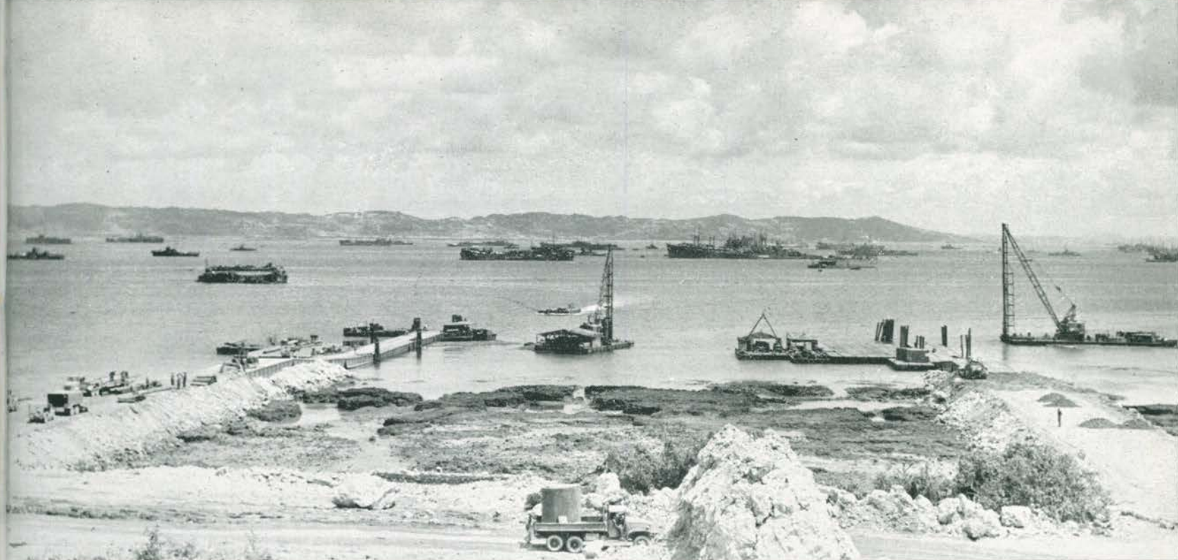
The approaches neared completion
