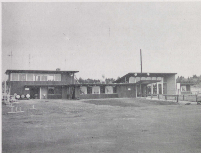
BANGOR STAYS ON THE AIR MAP Administration Building of the Bangor Municipal Airport at Old Town, designed by Eaton W. Tarbell and Associates.
