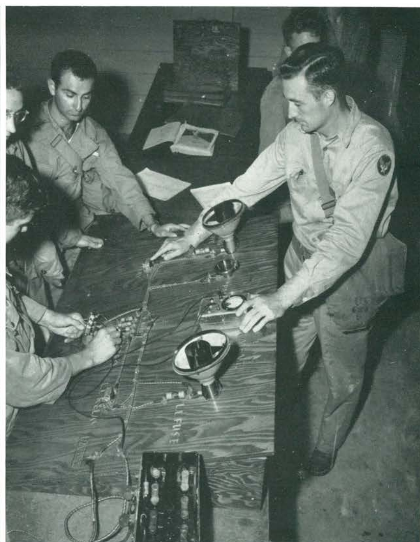
Explaining Electrical Blueprint.
