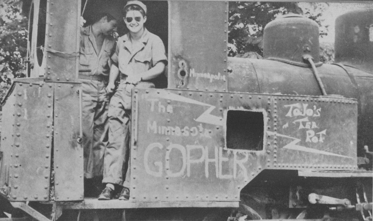
Monotony of steady work was broken from time to time by brief exploration trips around the island. Bob Blankenberg is shown, above , in the cab of one of the engines of the narrow-gauge railway system formerly used by Japanese to haul sugar cane. Below , Lieutenants Grow and Turner pose by a wrecked Nip tank in a jungle battlefield.
