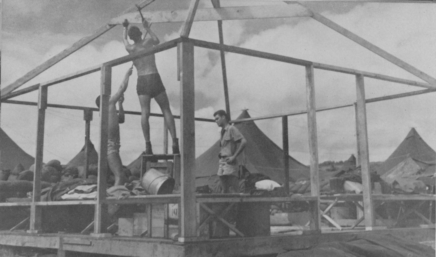
Construction went on at a rapid pace with the building of wooden frames for tents and the erection of Quonset huts for the coming combat crewmen. Maxwell, Pallas and Williams are shown above. Lower photo is of the sawmill, then located in what was later to be the motor pool area.
