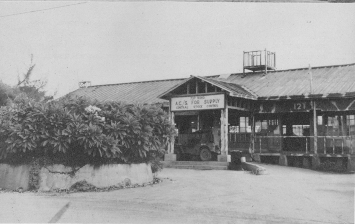
Some of the buildings used by Japanese garrison at Aslito (now Isley) Air Field were converted for use as offices and warehouses for B-29 units. Upper photo , Finance building. Air Corps supply, lower photo , occupies old Japanese Operations Building.
