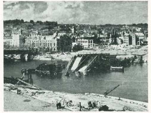
Bombed-out bridge, Rouen, France.
