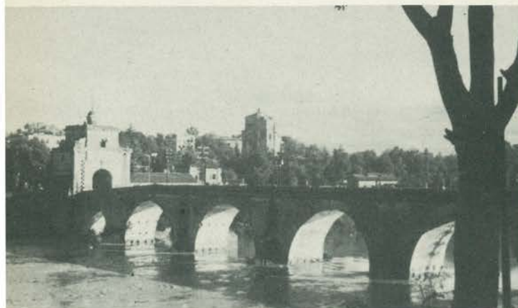
Pons Milvius: Rebuilt B. C. 109
