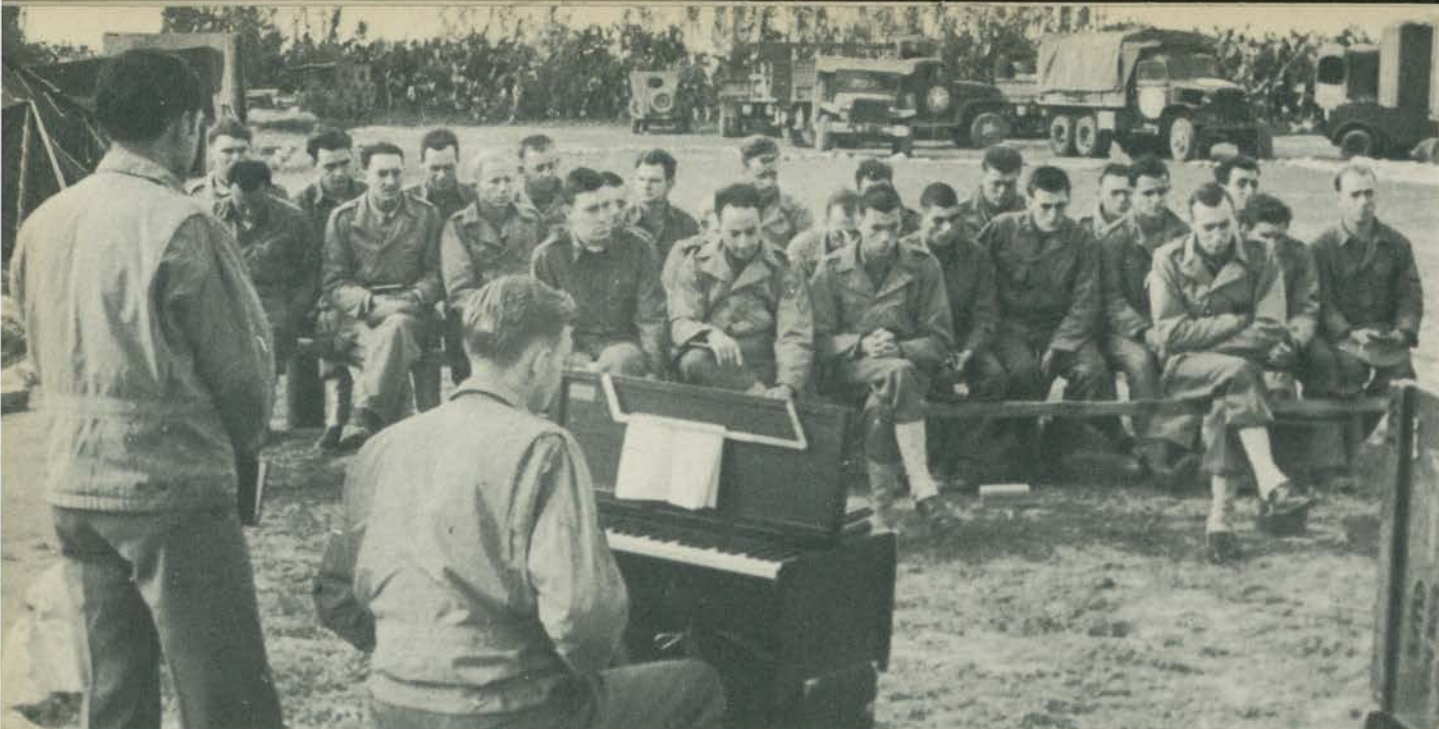
Service at B Battery
