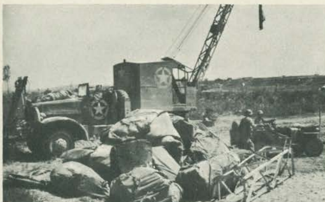
San Benedetto: First Step in Bridge Building
