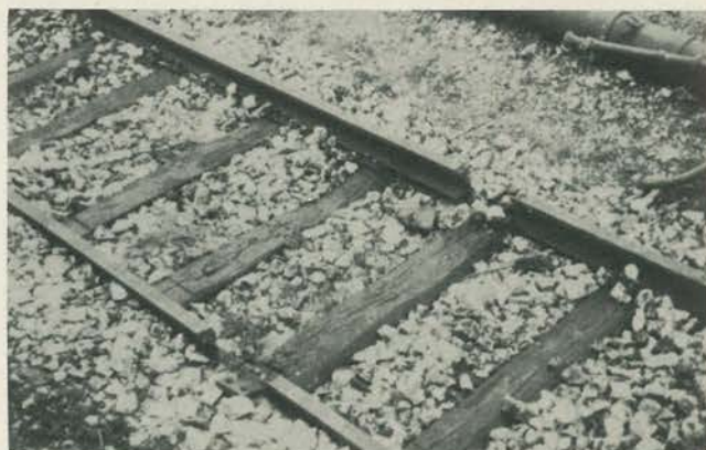
Near Rome: Railroad Demolition
