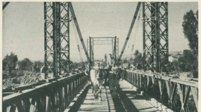
Near Florence: Experimental Suspension Bailey
