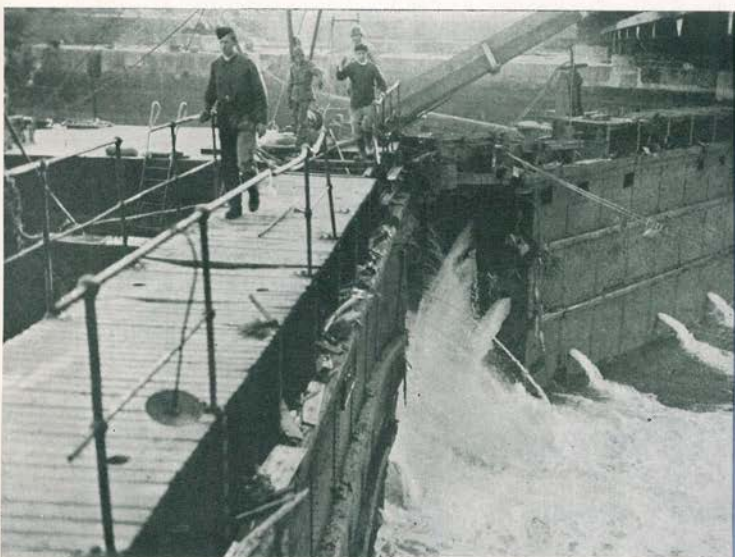
The Rochemont lock, key to Le Havre's inner basin system, was bulldozed into operation by Army engineers.
