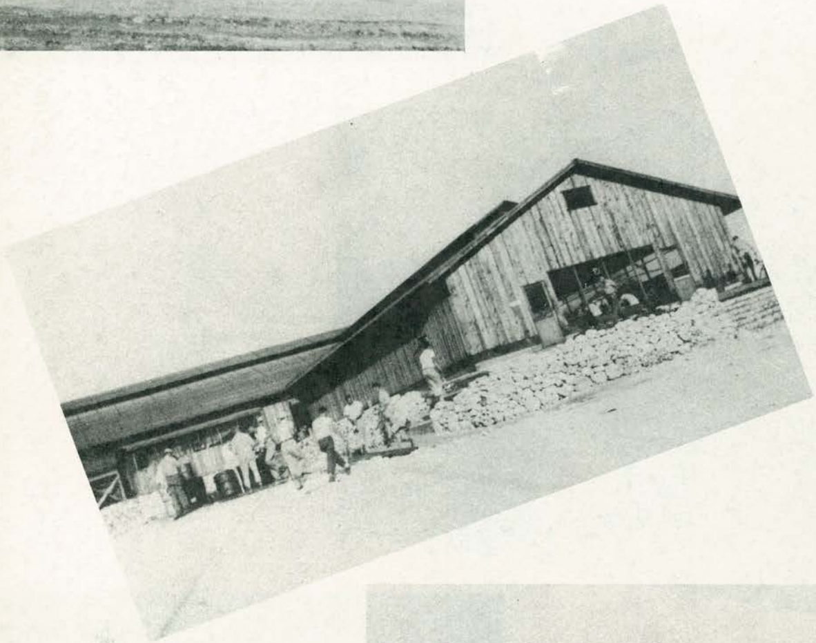
Mess Halls were completed
