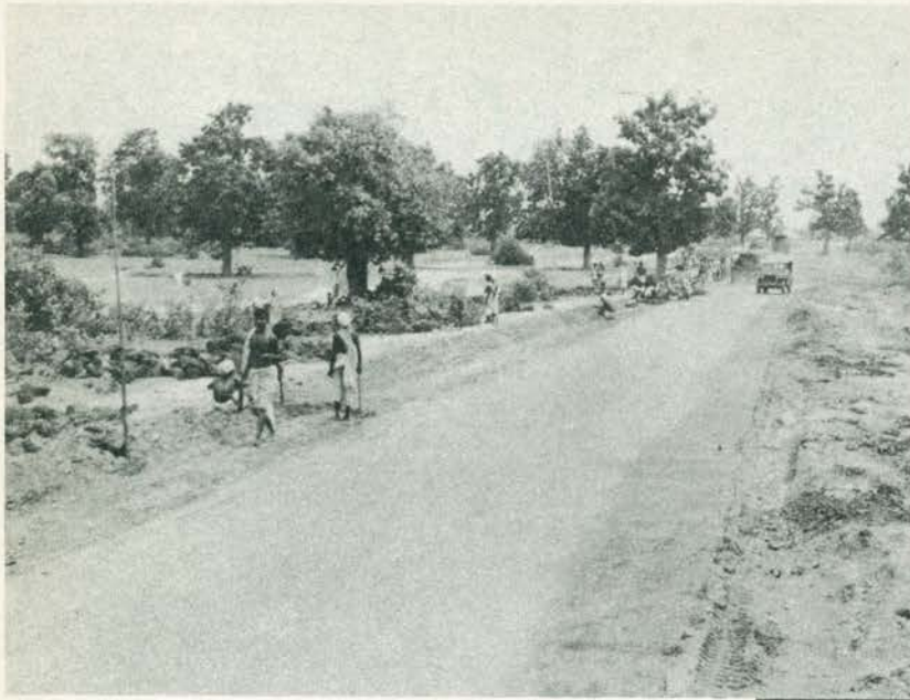
Road Repair Gang (110)
