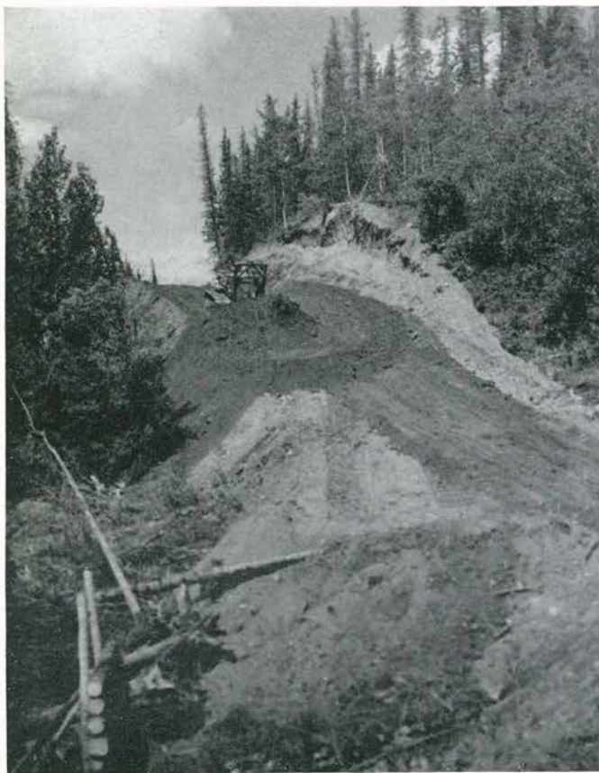
A dozer busy in a cut-and-fill job. An abundance of gravel nearby made short work of many otherwise difficult spots.
