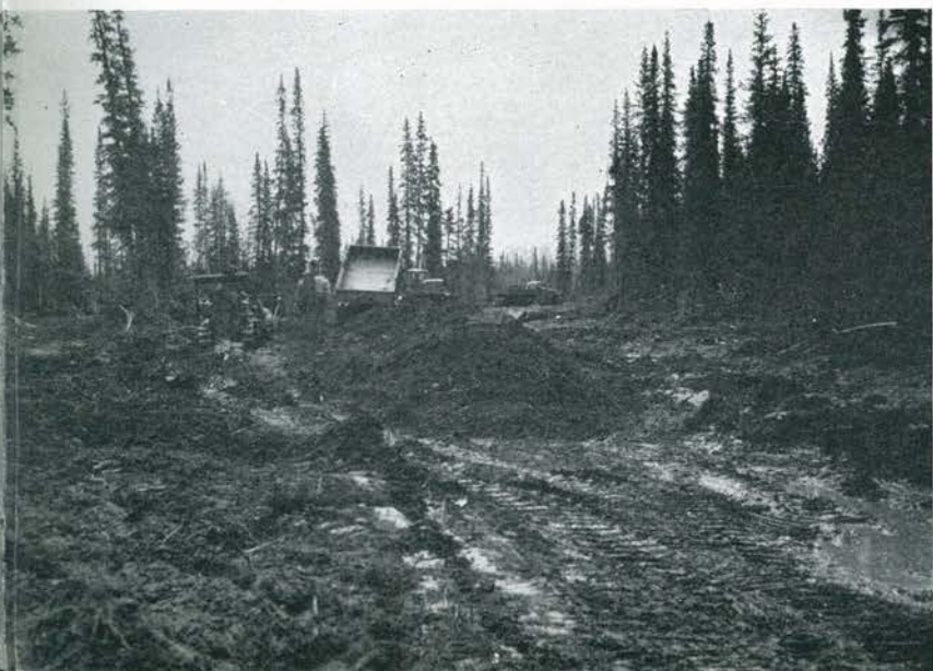
A Company's 1½-ton trucks graveling through swamp at mile 253, above Edith Creek.
