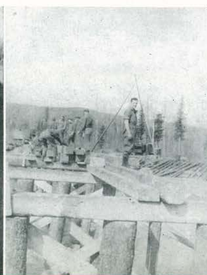
Stringers go down on log bents as C Company sets a fast pace.
