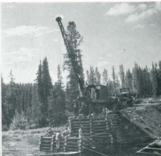
A mobile crane placing the footing for a trestle bent as D Company starts constructing the Morley River bridge at mile 26.
