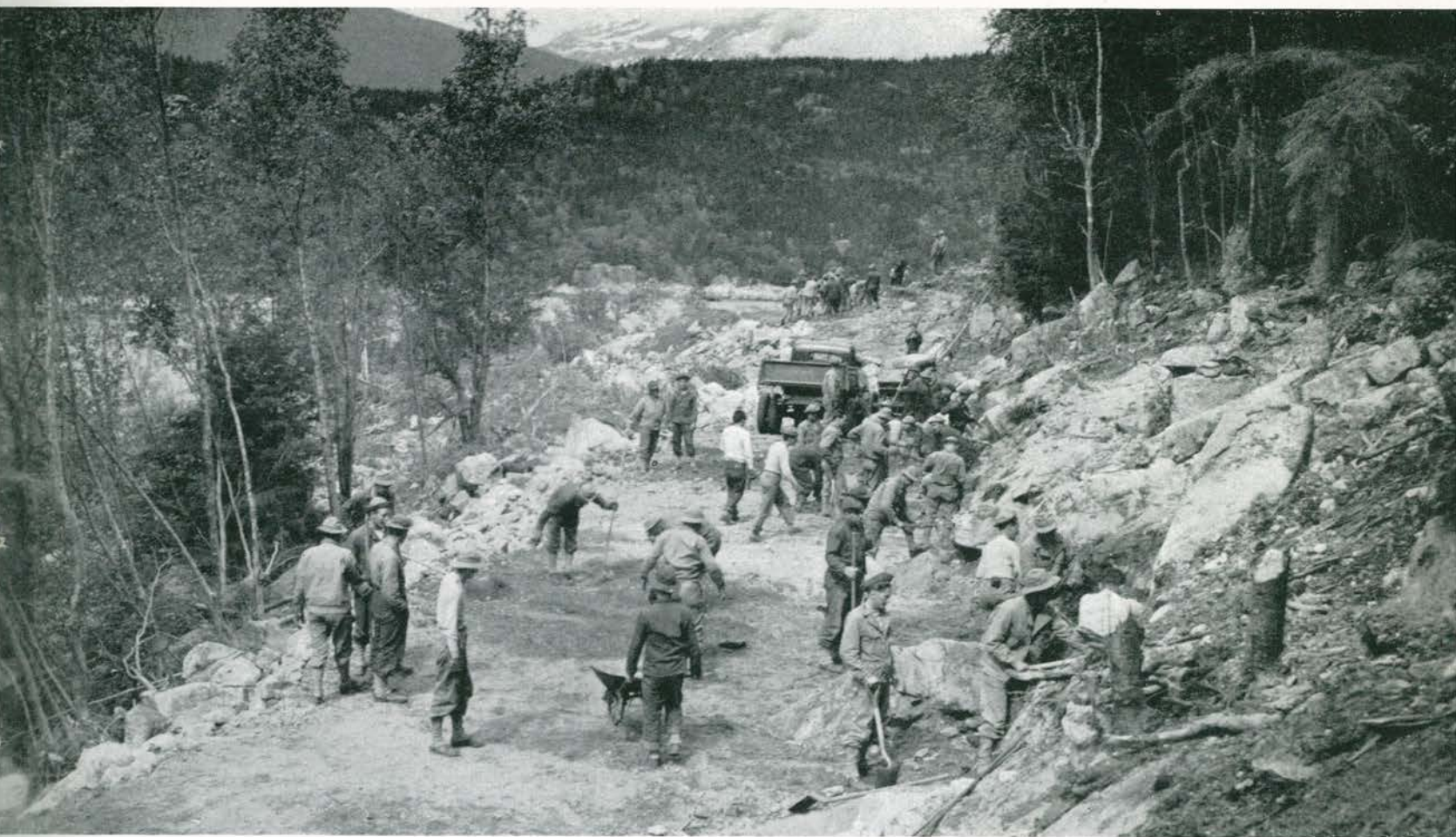
First Road Job—Skagway-Dyea—May, 1942.
