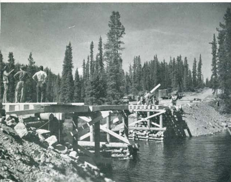
Only the center span stringers are yet to be placed as the Morley River bridge assumes shape. Flooring is already being laid.
