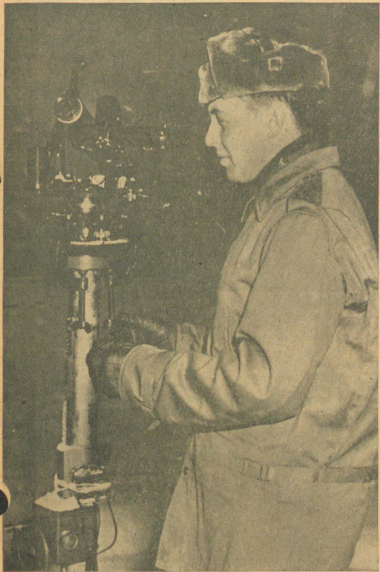
Theodolite at a Greenland weather station is operated during snowstorms. Small hydrogen balloons are released, viewed through theodolite to determine wind direction and velocity. Of the balloons released, many have been found and returned by Eskimos.
