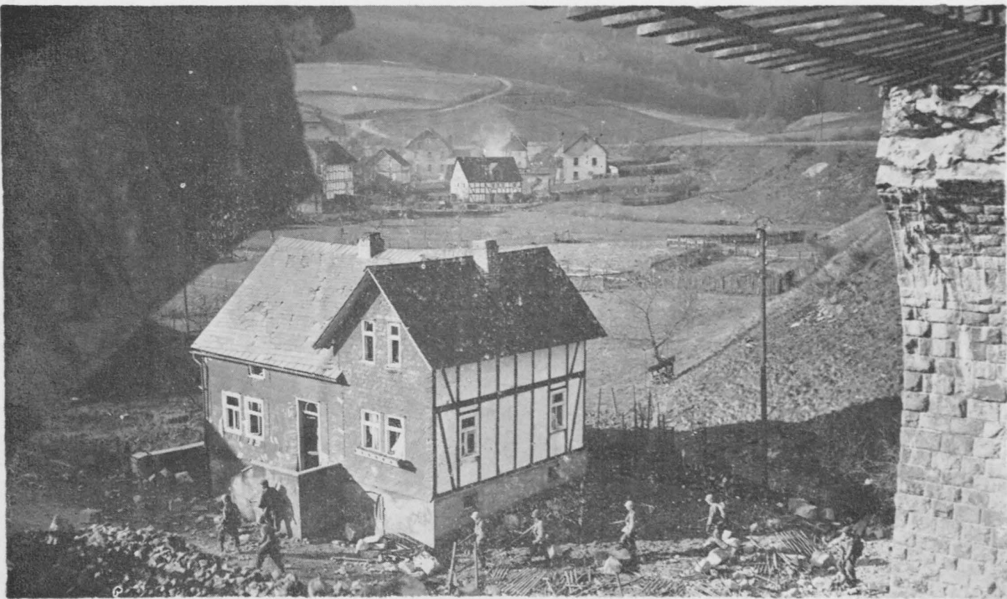
Near Olpe, elements of the 8th Division are shown advancing beneath a bombed railroad bridge. Minutes after this photo was taken, portions of the railroad track shown fell, injuring some doughboys.
