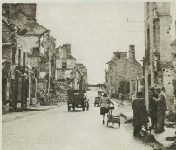
Laigle, France. Broken hulks of buildings on all sides gave mute evidence of the war's devastation.
