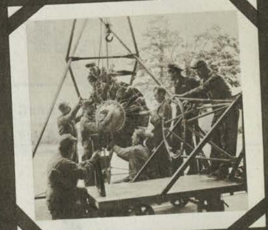
Engine mount designed by 67th Ser. Sq. personnel
