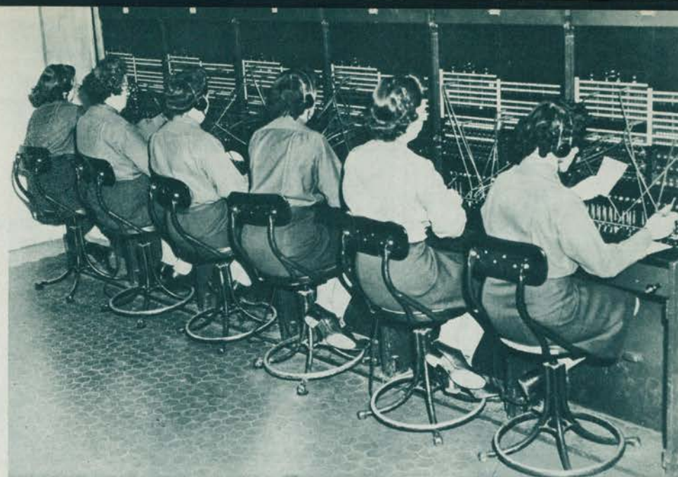
Eight thousand calls handled every twenty-four hours is the average achieved by the group of Signal WACs who operate the six-position switchboard at Command Headquarters in Creil, France.
