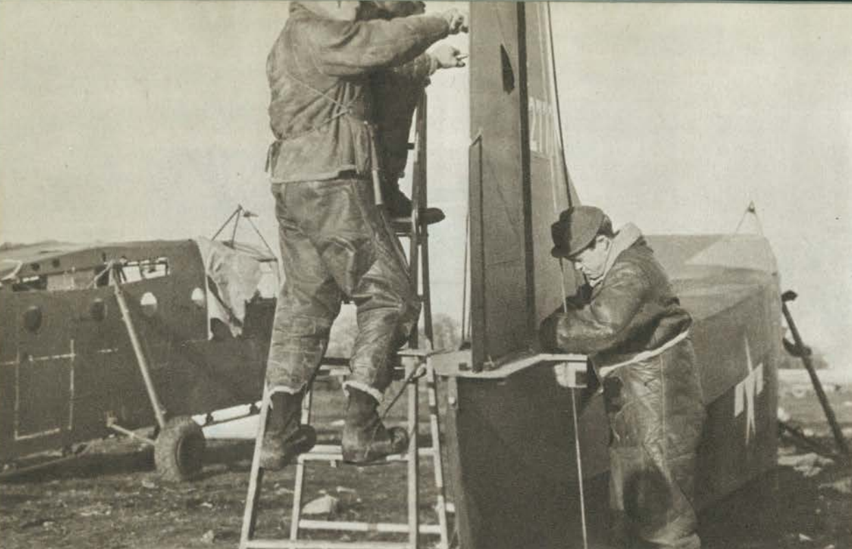
One of the first operations in assembly was the erection of the tail. Note heavy suits worn for weather protection.
