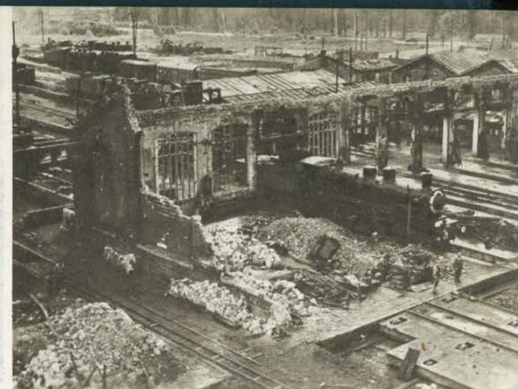
Battle damage at Creil was caused mainly by Ninth Air Force planes. Blasted locomotive shop testifies to accurate bombing.
