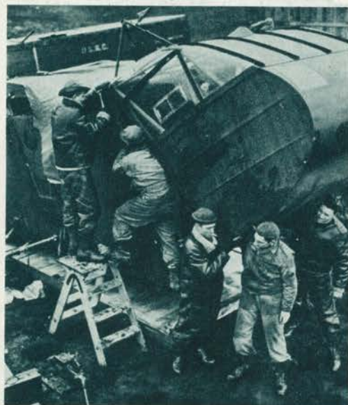
Assembling nose is a job requiring strong backs.
