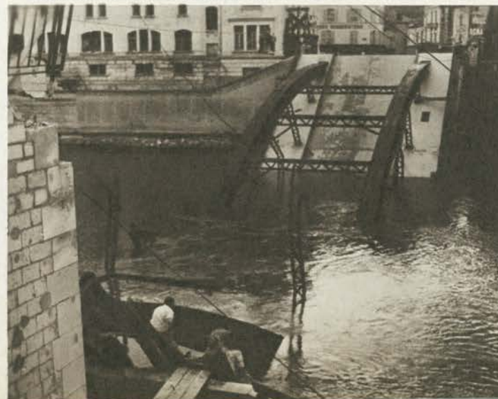
This bridge over the Oise River at Creil was demolished effectively by the retreating Nazis. A new pontoon bridge was built.
