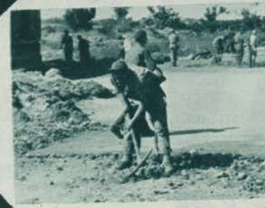
The pick and shovel brigade goes to work
