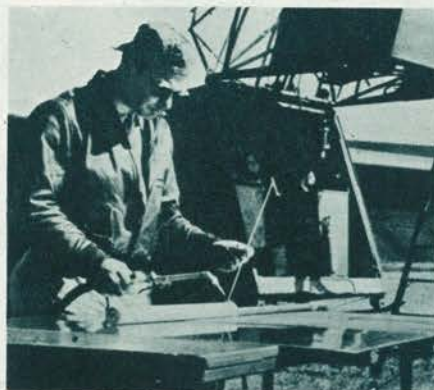
Sheet metal workers helped in the assembly.
