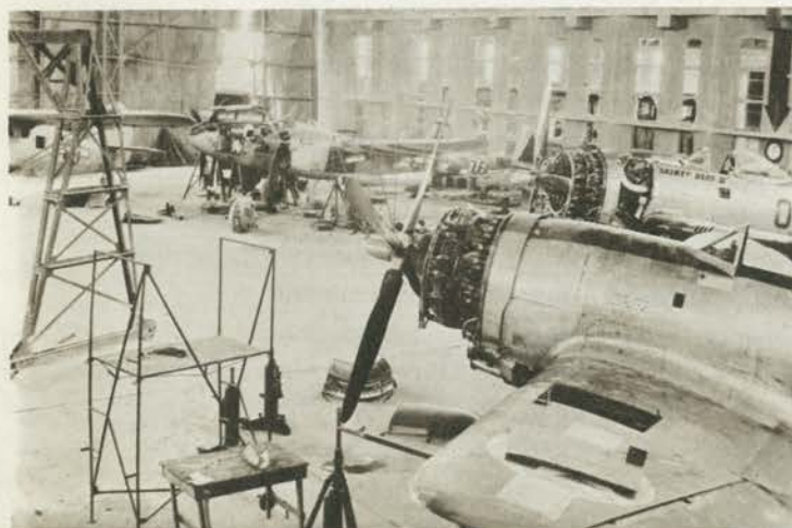
Most buildings on European airfields had been demolished by bombs. Fairly intact, this one became 74th Service Gr. hangar.
