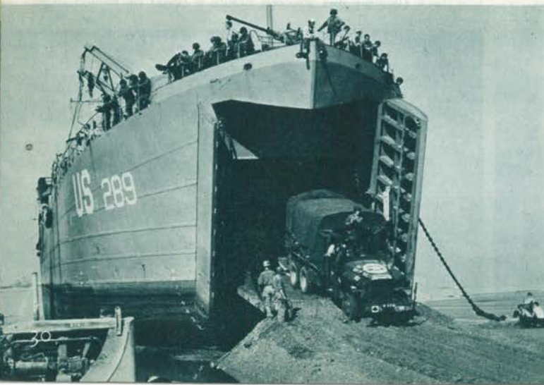
A truck of the 9th Service Group rolls from landing craft on to French soil. Note how sand is used to build roadway to boat.
