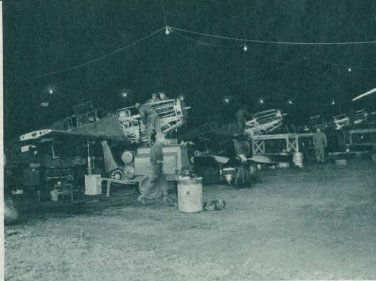
In a bulb-lift hanger, mechanics install the power plants of P-51s.
