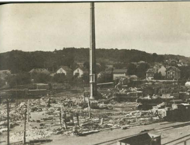
Through some freak of nature, this tall chimney stands quite undamaged among the bomb-wrecked marshalling yards at Creil.
