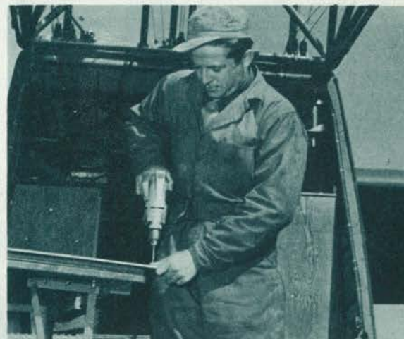
Mechanic is shown rivetting a part of the glider controls.
