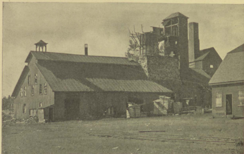
Old Furnace at Katahdin Iron Works.
