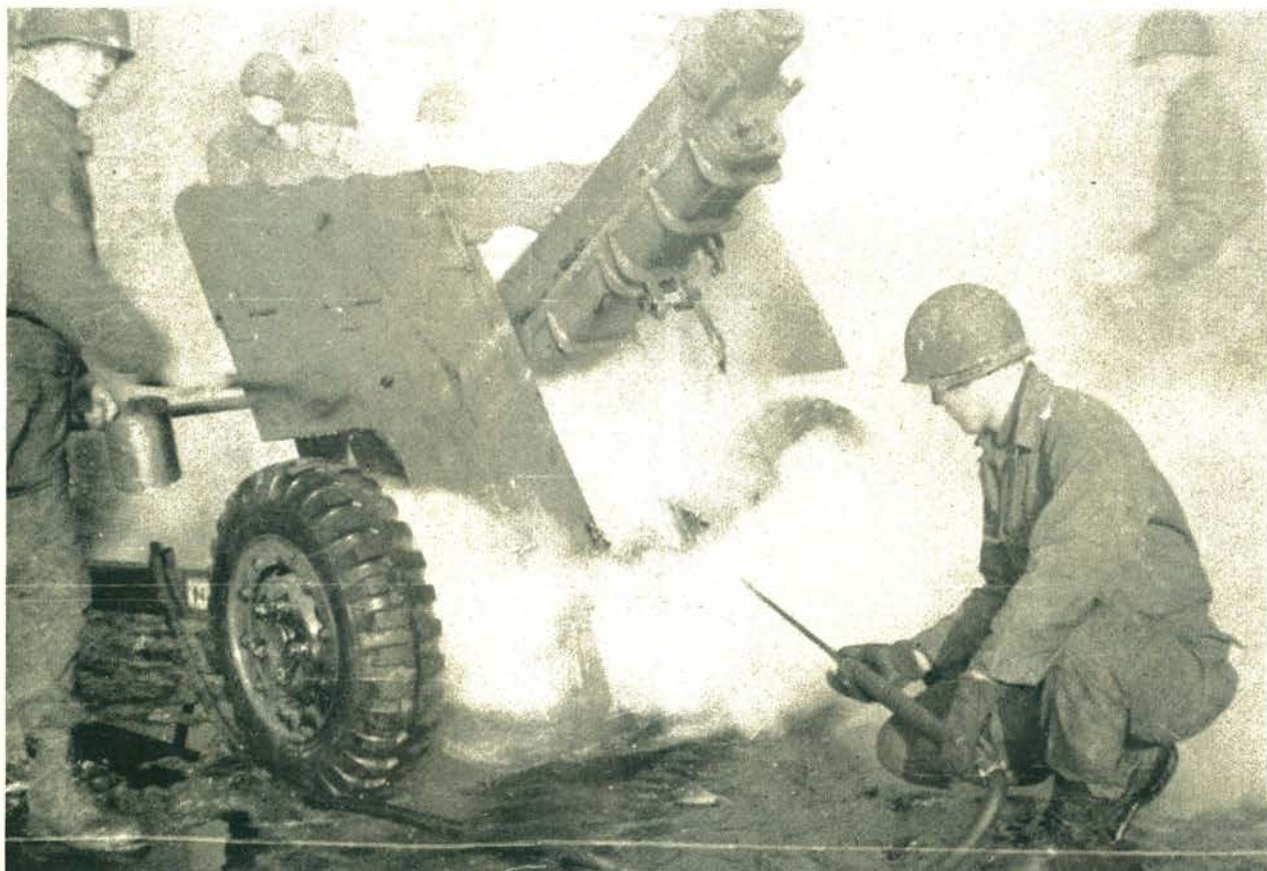
Steaming a 105-mm howitzer to remove all traces of the cosmoline with which it was coated prior to shipment overseas.
