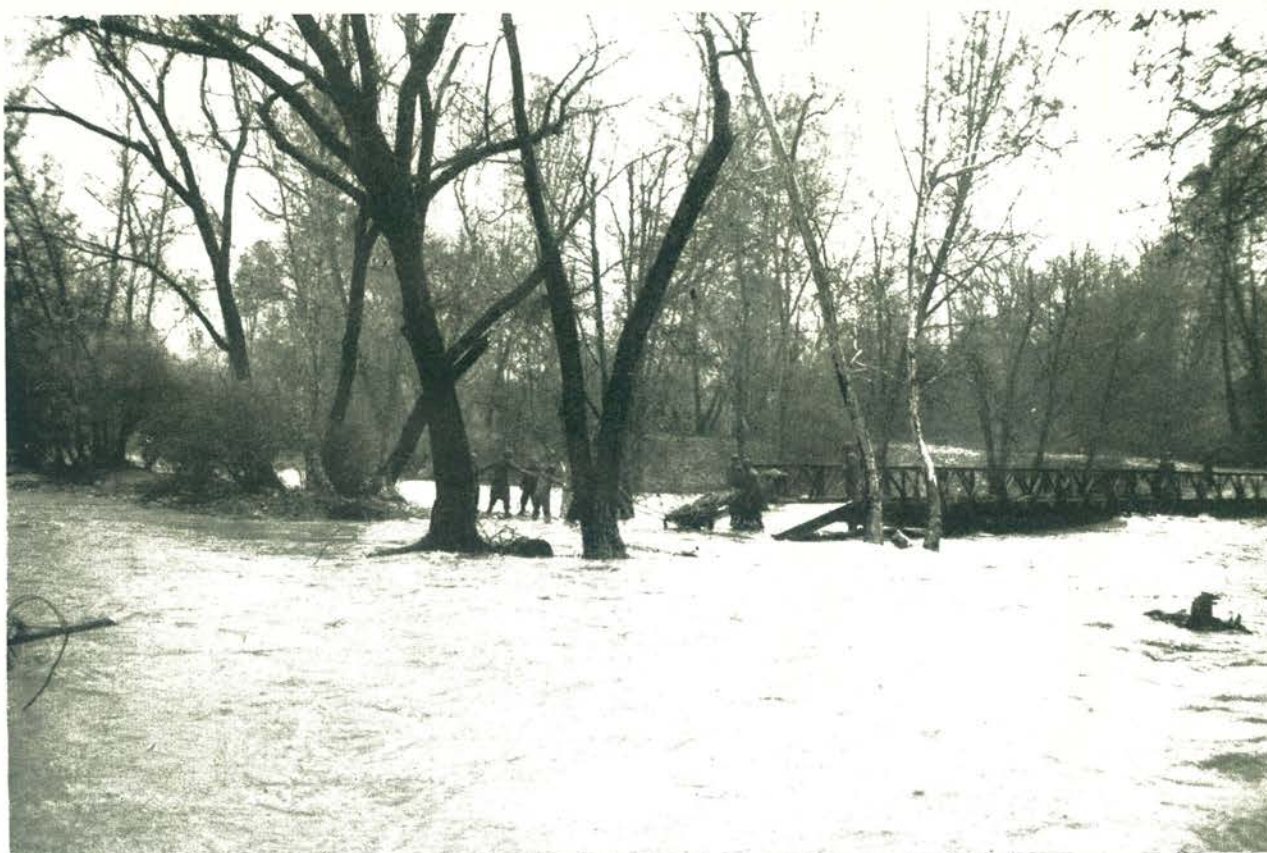
271st Engineer Combat Bn. troops lash a Bailey Bridge to trees to prevent it from being washed away by the flooded north fork of the San Antonio River during the Hunter Liggett maneuvers.
