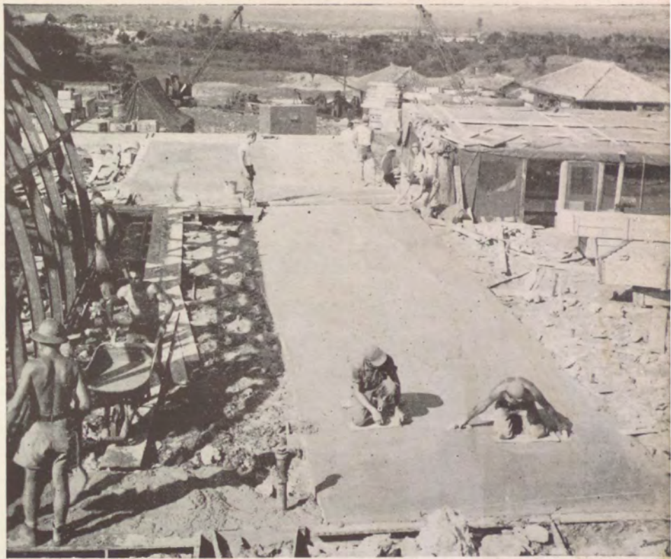
Finishing Concrete Slab for Reefers
