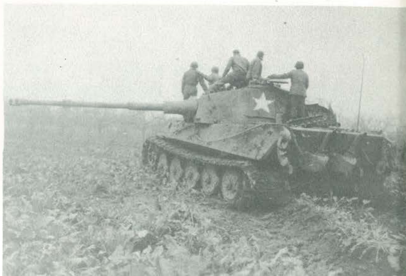
Captured German Tiger tank being moved out of a field by Ordnance men of the Seventh Armored Division, after repairs have been effected on the captured vehicle, which was taken near Gereonsweiler, Germany. (15 December 1944)
