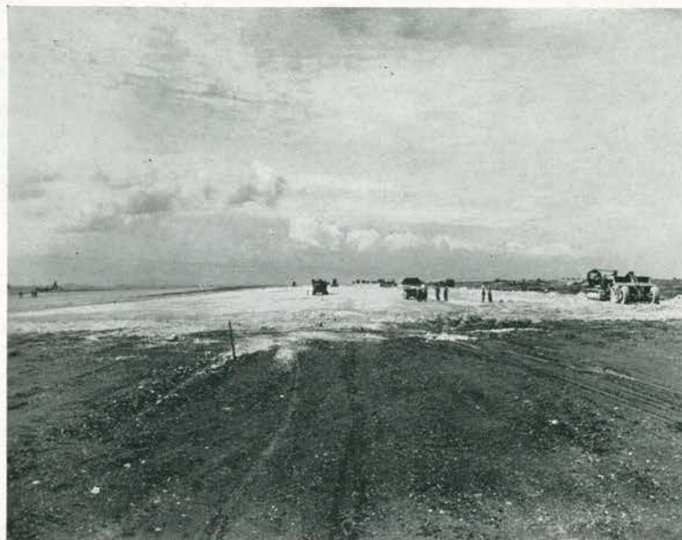
CONSTANT RAINS have turned sub-grade into a bog. Pans have been brought back to work over the wet coral. All finishing work is practically at a standstill, but the gang is loading chunks of rock removed from surface to utilize time.
