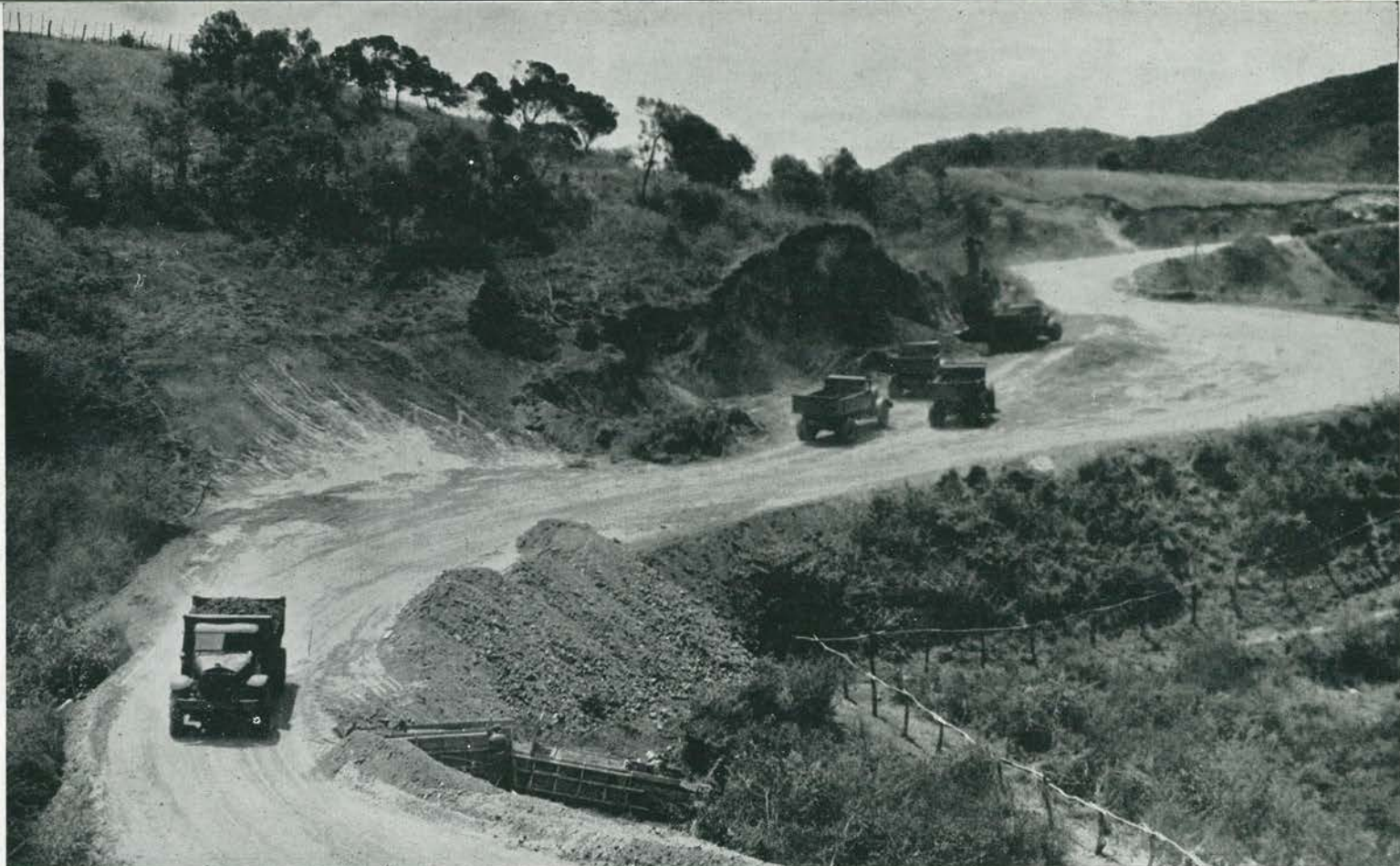
LITTLE BURMA ROAD. Snaking over exceedingly treacherous mountain passes, the original road above Bourail was actually no more than a narrow 15-foot wagon trail. Earth, cut away from the bordering red-dirt bluffs, was dumped over edge on opposite side
