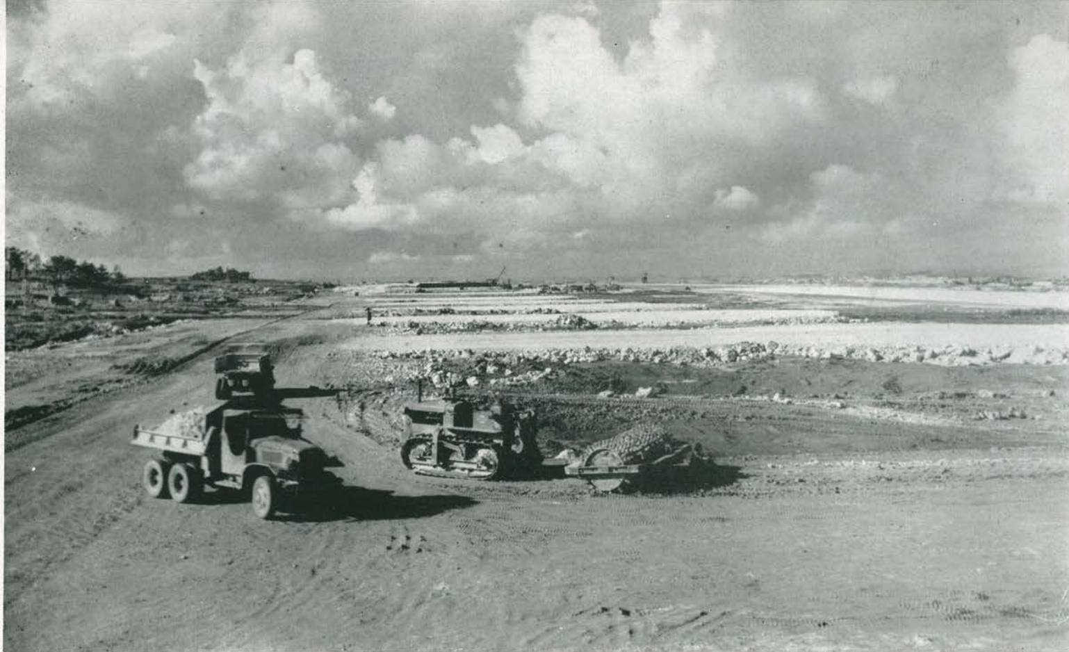
COMING AND GOING. An empty truck heads back to the pit for another load of coral as a full vehicle turns into a hardstand to dump its burden. This is a general view of unpaved taxiways and paved hardstands looking south. Bolo Field proper is at right. Sheepfoot roller (foreground)
