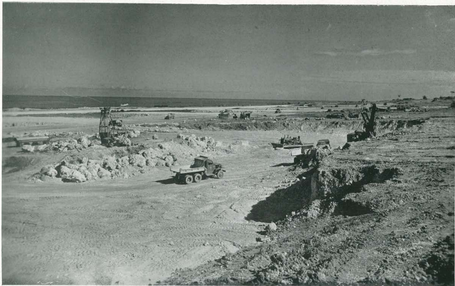
CUTTING ON "C" taxiway goes ahead as pans cut out adjoining hardstands on taxiway east of the completed runway. Most battalion equipment has been moved to this new location. To the right of light tower are a few remaining piles of asphalt barrels. A roofer, pulled by 'dozer (right center), softens up the cut for pans. Tails of the new Douglas A-26 attack bombers (far right) are barely discernable. The taxiways at right are already completed and ready for occupancy.
