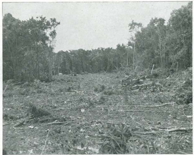
AND DAY IS DONE. The end of the first day. An area of 300 feet in width and 600 feet in length has been roughed clear. A good, fast start on a good fast job—on the road to Tokyo! However, the 87th was to build many more strips before V-J Day.
