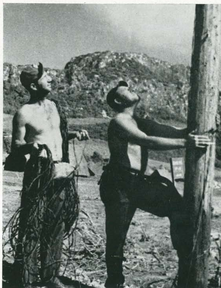
WIRED FOR ACTION. William Shady (left) "gets a line" on pole as Andrew ("Mule") Steadley prepares to mount native timber. Altogether, 50 miles of telephone and 20 miles of electrical wire knitted the staging camp into a tightly-woven unit.
