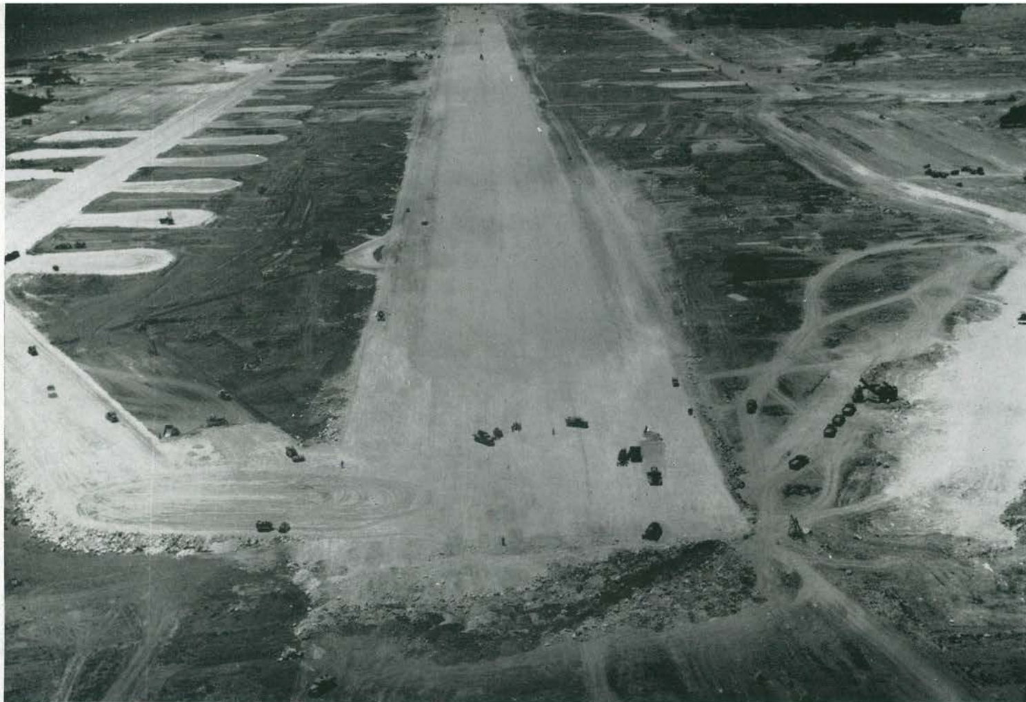
HEAVYWEIGHT! Close-up aerial of Bolo Field, still under construction by 87th Seabees, shows airfield makers and equipment rushing to finish sprawling B-29 strip in time to help deliver knockout blows to hard-pressed Japan. Jackhammer crews remove niggerheads (central fore-
