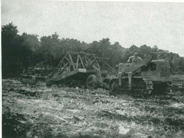
SKIMMING OFF THE MUD. Before grading the runway to shape, it was necessary to clear off the black humus overburden. Here, two HD-10s struggle to load an eight-yard pan with the sticky muck shortly after a terrific downpour.
