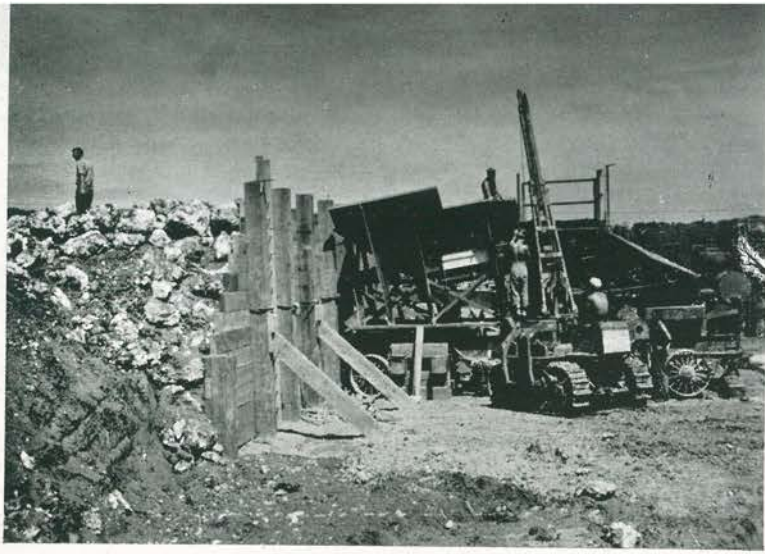
FIRST UNIT of the rock crusher assembly at Nagahama Quarry is being erected as the jaw crusher is set in place. Heavy timber bulkhead, set against formidable earth ramp (left), provides an easy approach for rock-laden trucks.
