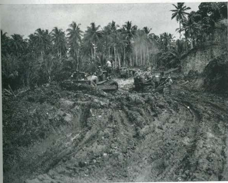
MUD. Even giant bulldozers sometimes bog down in tropical mire. Here, Tom Hutson rescues "Chet" Wlostoski and his stuck 'dozer from the muck. Huge fills in swamp made this road project a stiff proving ground for both men and equipment.
