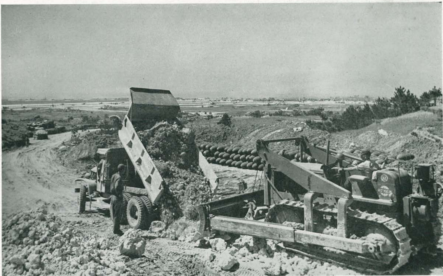
IN THE DUMPS, "Kask" Conine dumps a load of rough coral on newly constructed access road into Yontan bomb dump as Meredith Walls (standing, left) checks grade. Oliver Autry (right) operates the 'dozer. A pile of 500-pound aerial bombs stacked in the revetment may be seen, in part,
