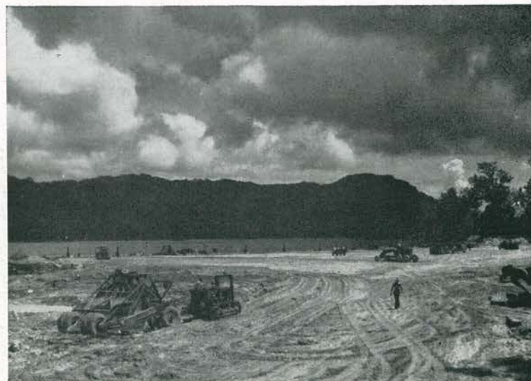
HILL DISAPPEARS. Grading of the cleared dock area is now progressing by leaps and bounds. The hill, which formerly was here, has been carved away and used as fill on shore access road. Plane tender is anchored offshore with PBVs.
