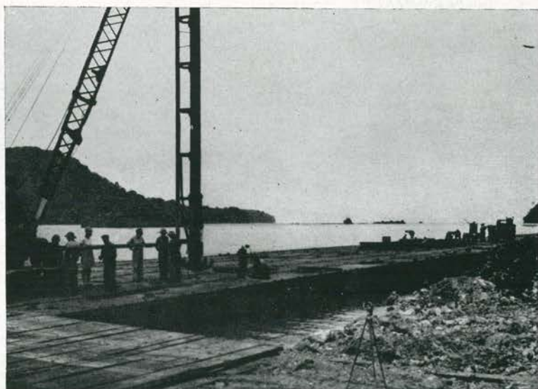
PILE-DRIVER rig is poised to sink one of many piles used for dolphins and clusters. Piles were sharpened and steel-tipped to secure them in coral bottom. Net tender and barge (right) are laying submarine net across harbor entrance.
