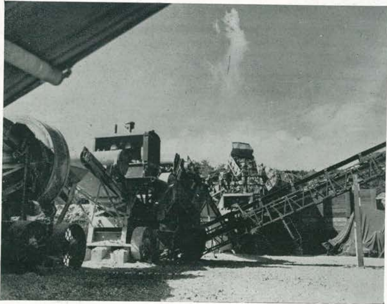
THE WORKS. Here is an overall view of entire unit in operation from time rough rock is dumped into crusher (center) until it is carried up conveyor belts ready for use. Nearby quarry was considered a dangerous assignment.
