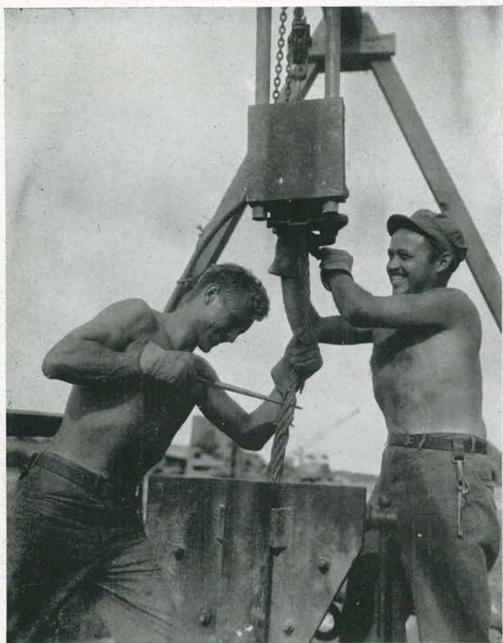
GENERAL RIGGING LOFT handled all assignments not pertaining to transportation equipment. Fred ("Buttercup") Haas (left) belies his nickname as he executes a neat splice on a heavy cable. Tutor John ("Pinky") Doyle smiles down proudly upon his protegee.
