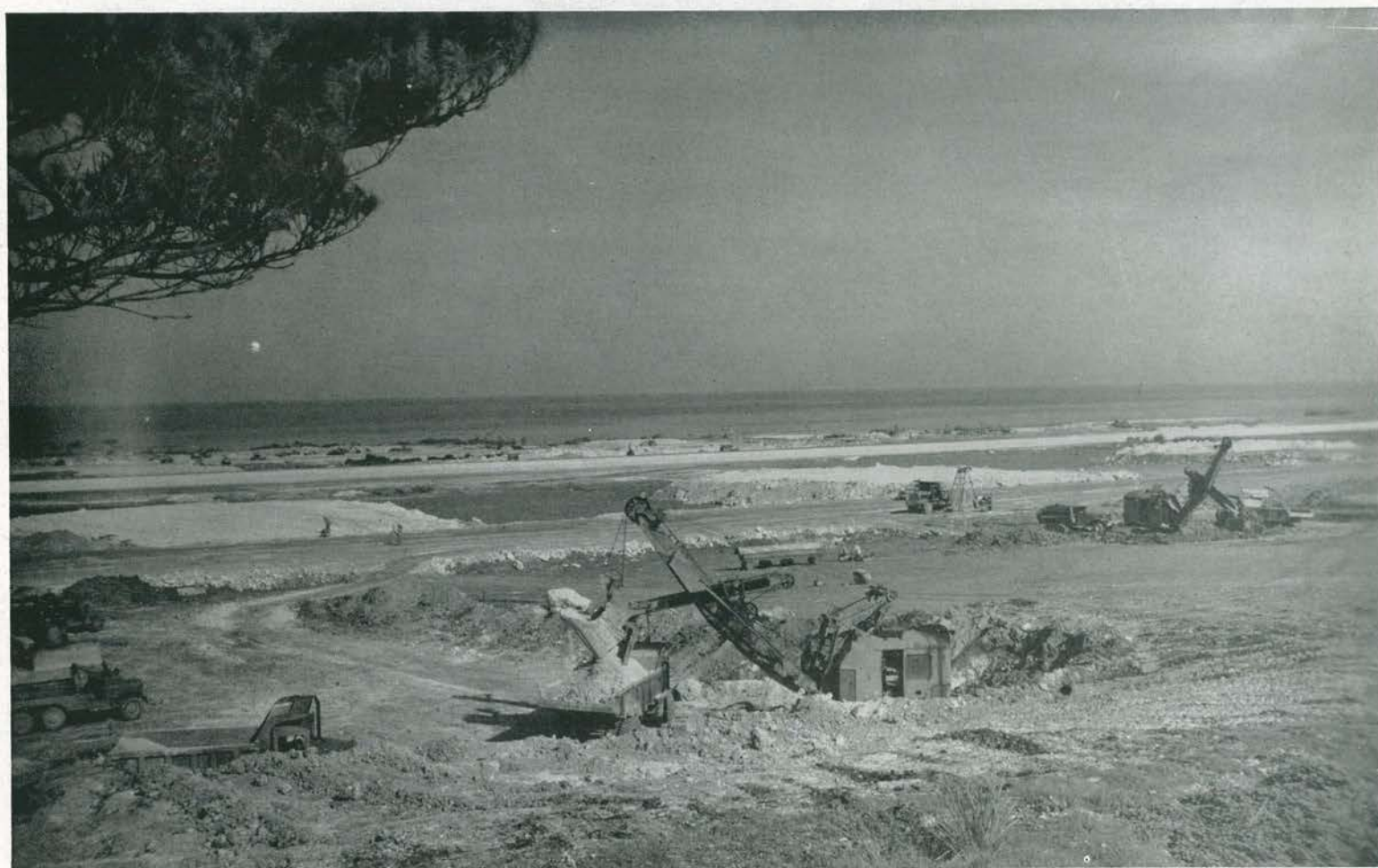
LOOKING WEST across Bolo Field to the East China Sea, a 2\frac{1}{2} -yard shovel loads a Euclid with one of last loads of coral used. A 1\frac{1}{2} -yard shovel (right) digs dirt out of last hardstand. In 1943-44, Stirling Airfield
