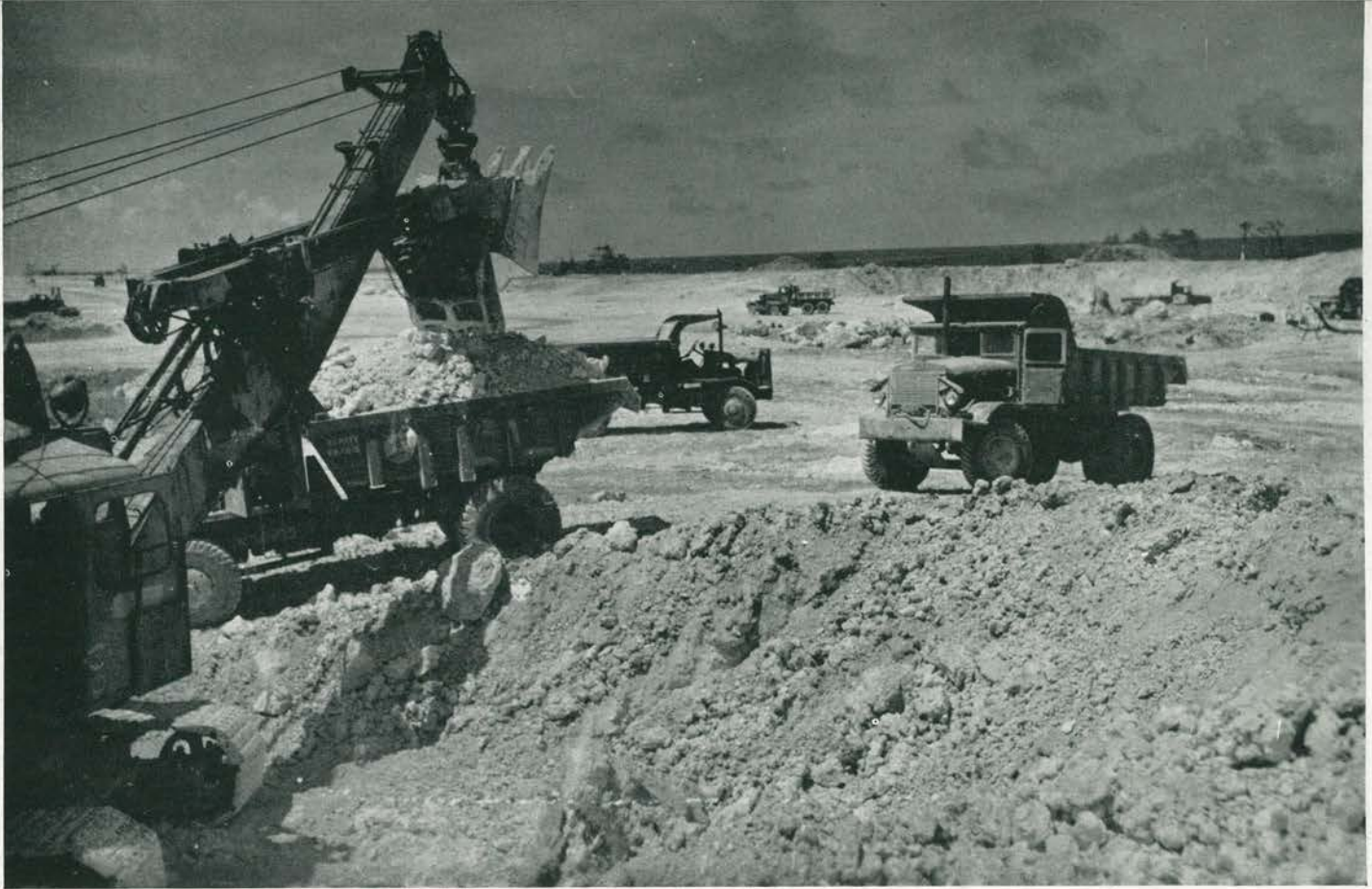
BIG PIT. A 2½-yard shovel and a small fleet of Euclid trucks are working out huge portions of coral at spot known as "the big pit." This site supplied coral for most of runway, plus connecting link with west taxiway.
