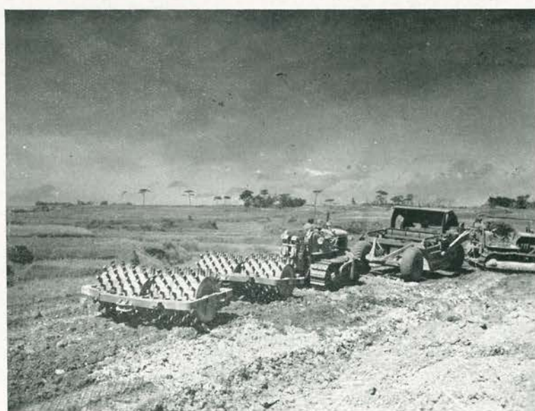
AT LAST. Actual work on Bolo Field commences on 19 June after many false starts and the 87th's last direct contribution toward winning the war is under way. Here, sheepfoot roller compacts fill behind 12-yard pan.
