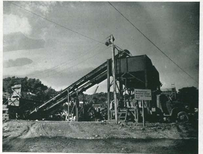
STORAGE BINS for crushed stone (right) feed materials into trucks that haul it to various projects. These bins are filled by means of conveyor belts (left), which are driven by crusher motors. No unauthorized personnel were allowed.
