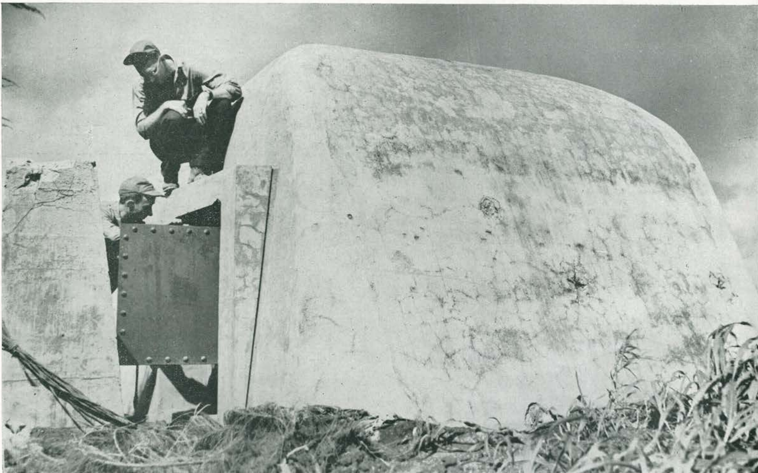
JAP PILLBOX. Numbers of these formidable fortifications still rimmed the future B-29 field after invasion—an ignoble monument to short-sighted Jap stupidity. These pillboxes, constructed of reinforcing steel and concrete three feet thick, were apparently impregnable to attacking troops. Two
