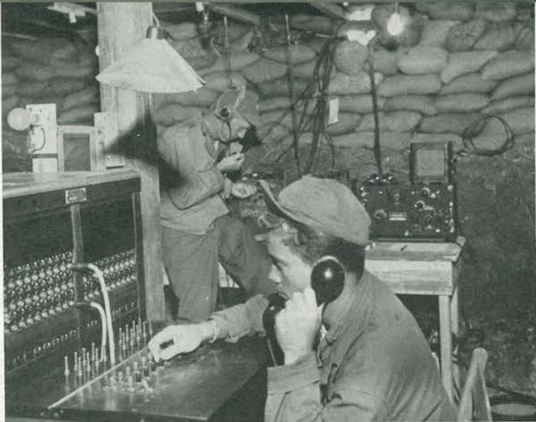
NUMBER, PLEASE! John Hatcher (foreground) puts through first call on switchboard in new underground communications center as Lieut. A. L. Davis, E Division Officer, tests radio set. Constructed of sandbags, Jap rails, etc., this structure proved invaluable.
