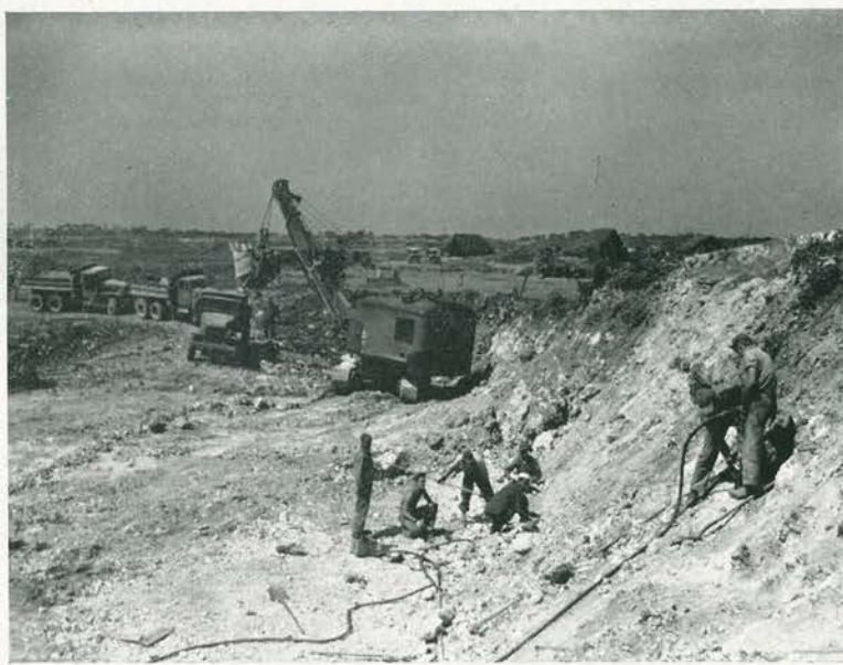
GRAND OPENING. A power-shovel starts cutting into one of the two coral pits that are to provide all paving material for the Bolo job. Demolition gang drills hole for charge to loosen up solid portions of the coral formation.
