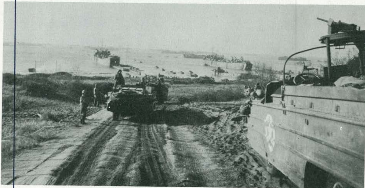
MEN AND EQUIPMENT COMING ASHORE AT ANZIO
