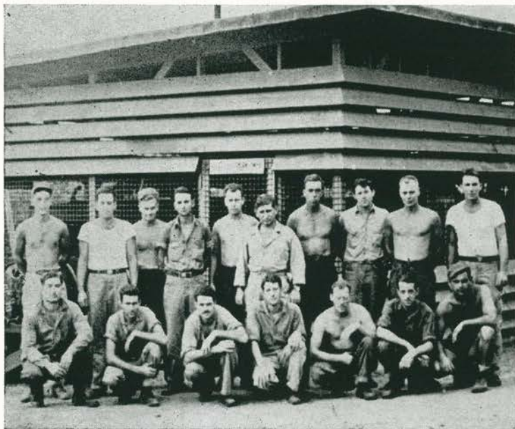
CHIEF WALKER'S ELECTRICAL CREW
