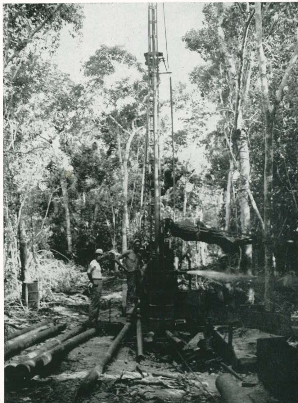
DRILLING A WATER WELL
