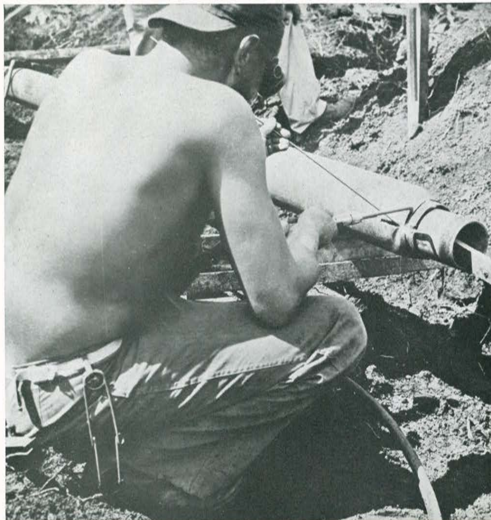
WATER LINE WELDER
