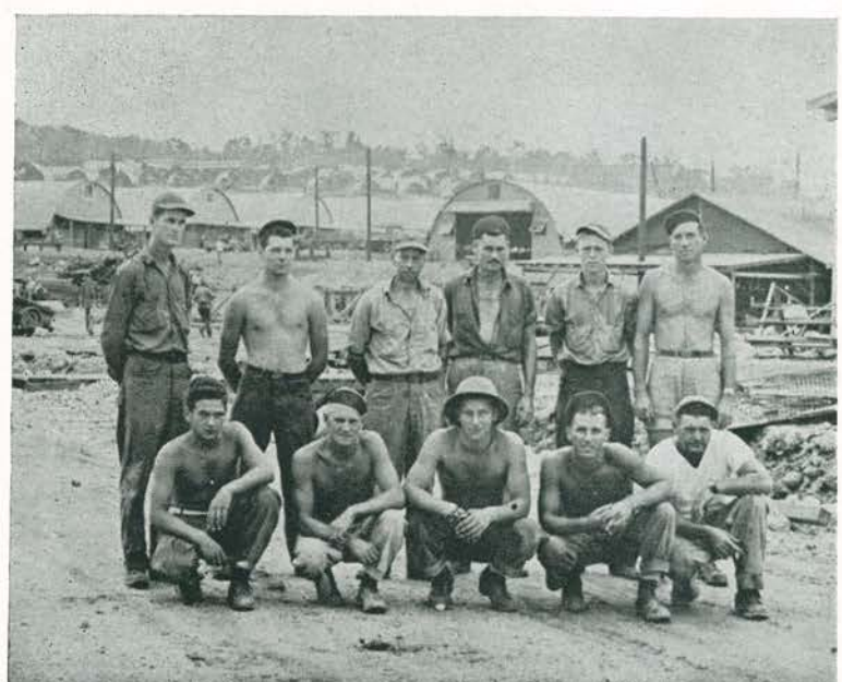
CEMENT FINISHING CREW
