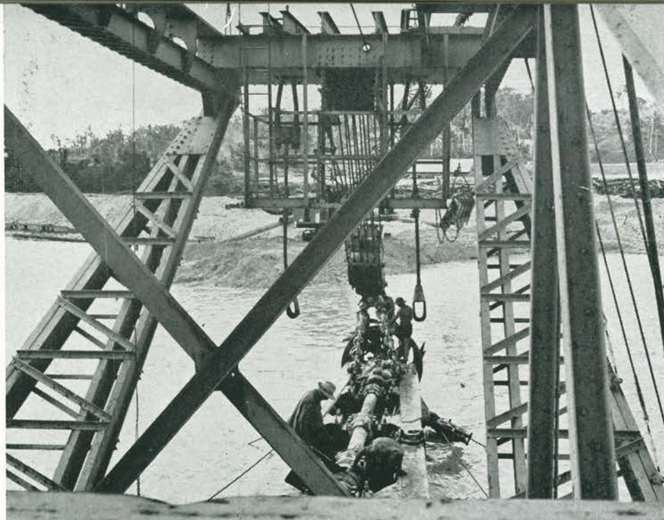
DREDGE SUCTION AND CUTTER HEAD
