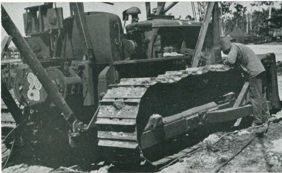
WELDING ON A D-7
