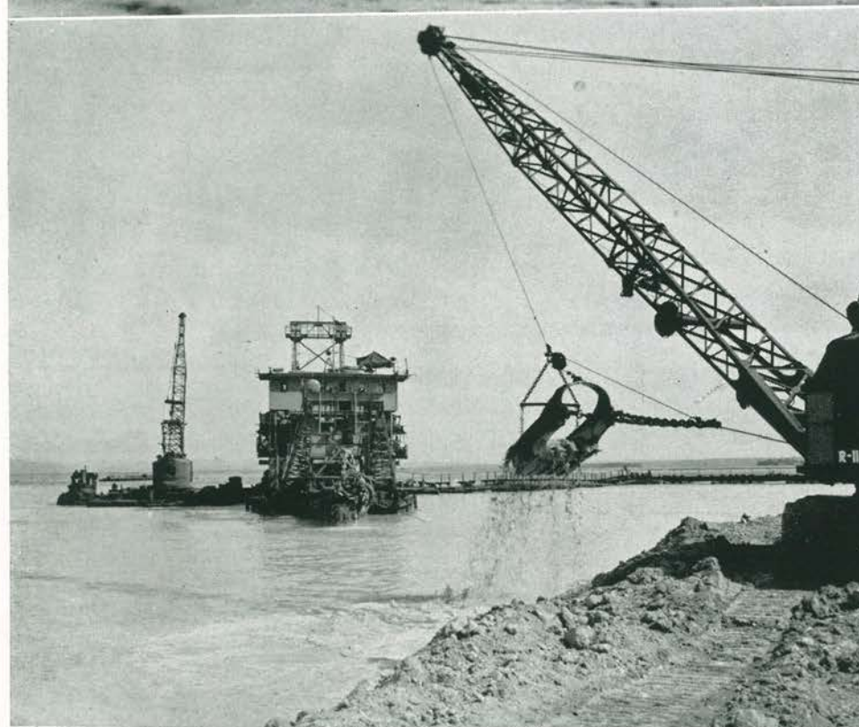
SUCTION DREDGE IN OPERATION
