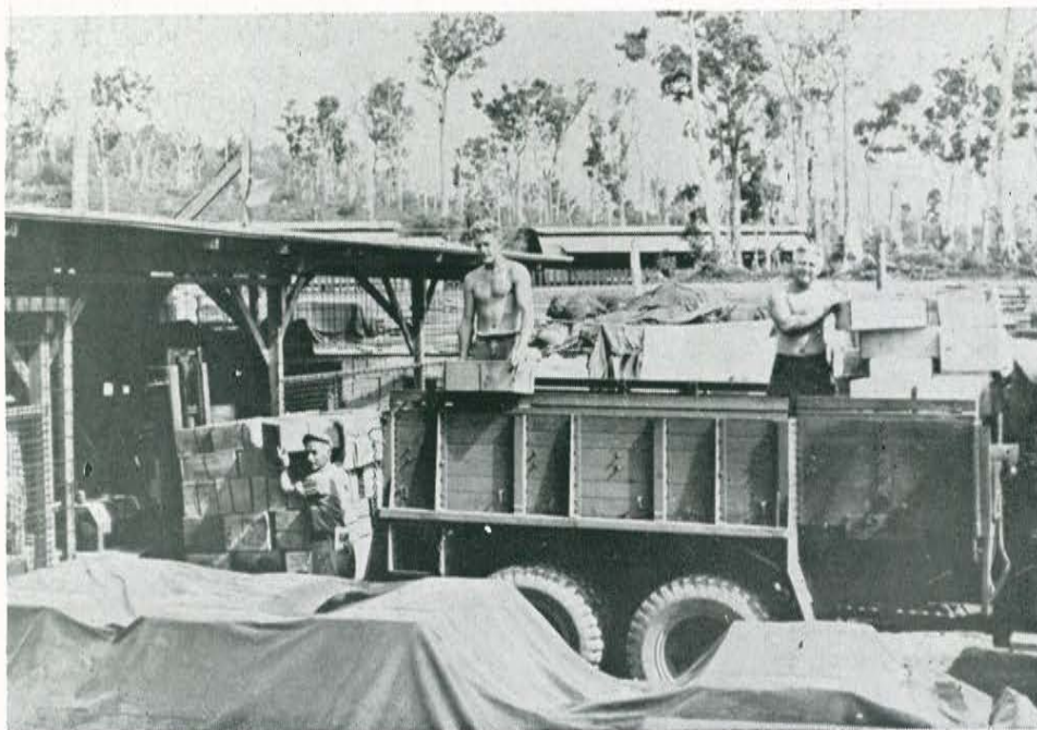
UNLOADING OUTSIDE OF WAREHOUSE
