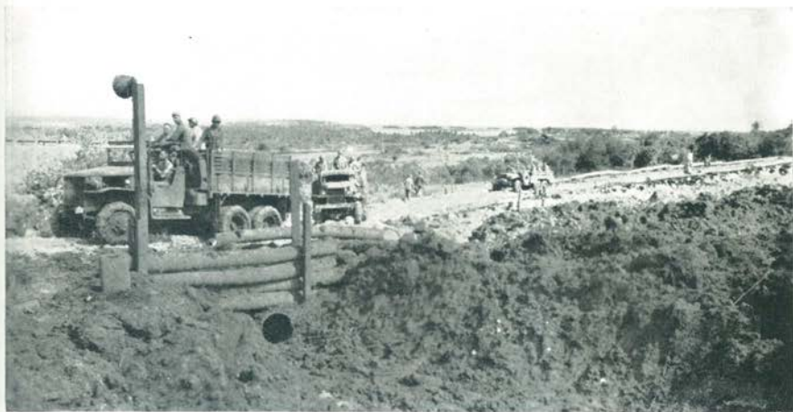
Johnson Road was completed.
