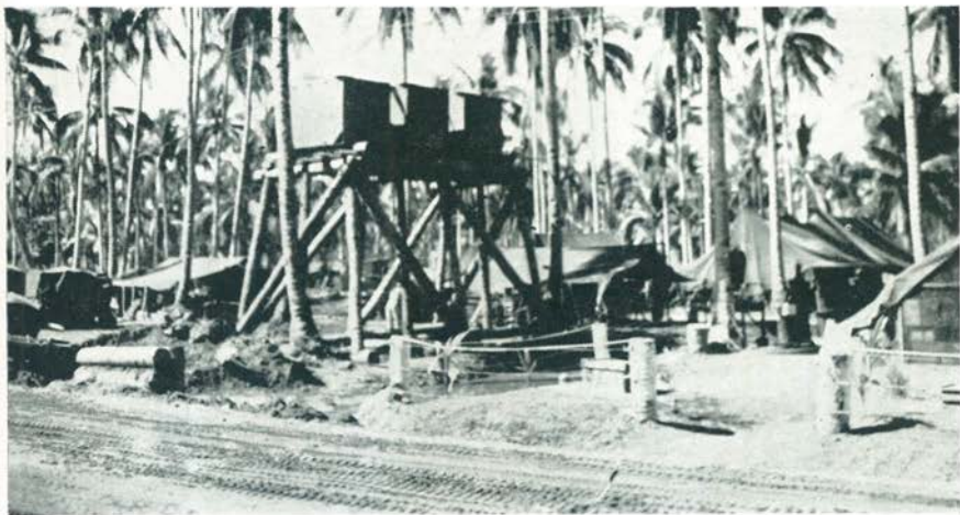
Running water to the company kitchens.
