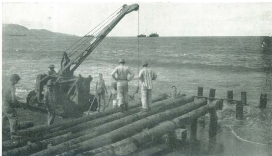
The new job was that of constructing ten coconut-log piers.
