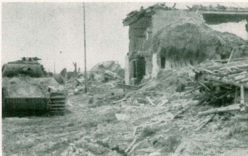
"the piles of rubble"
