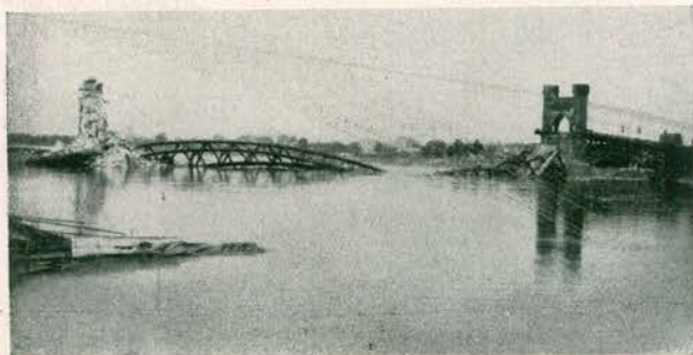
RHINE BRIDGE AFTER COLLAPSE
