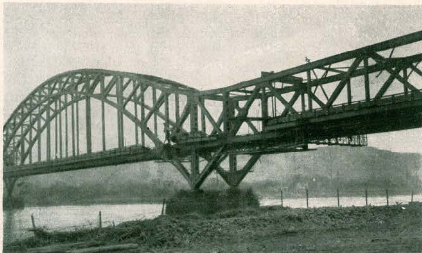
EAST END OF REMAGEN BRIDGE BEFORE COLLAPSE
