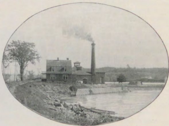
BANGOR WATER WORKS.
