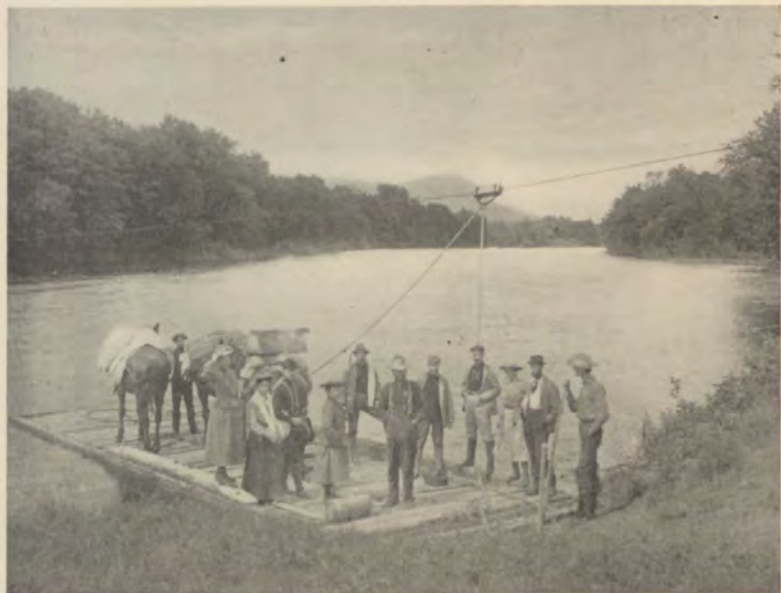
The East Branch Ferry.
