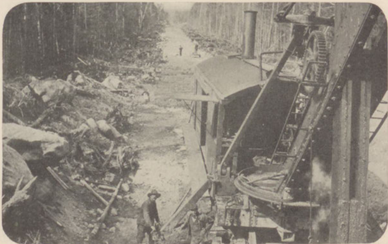
AT WORK ON THE MEDFORD CUT-OFF.
