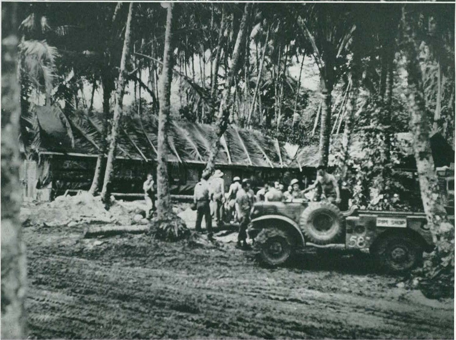
58 th C.B.'S STRIP WORKERS MESS HALL •
